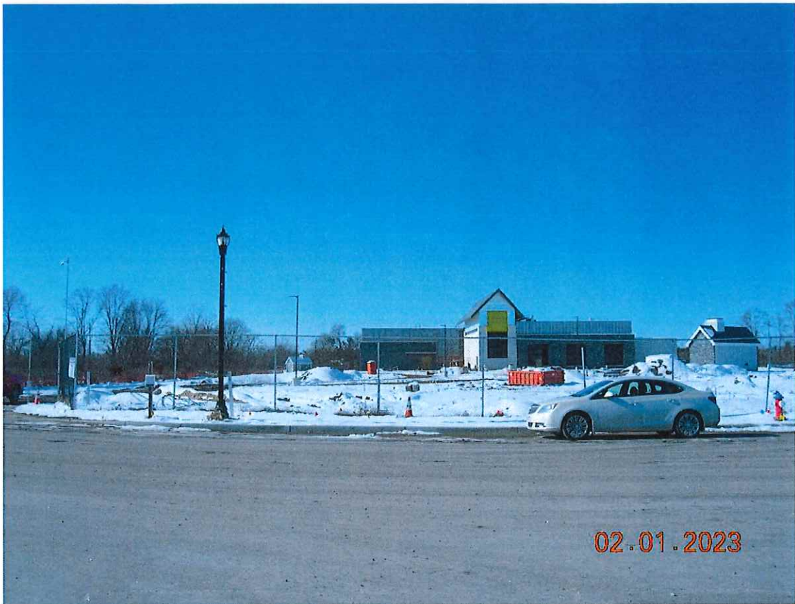
P1. Looking westerly from the current Veterans Parkway terminus / cul-de-sac toward Lot A and the city water production and treatment facility currently under construction.
