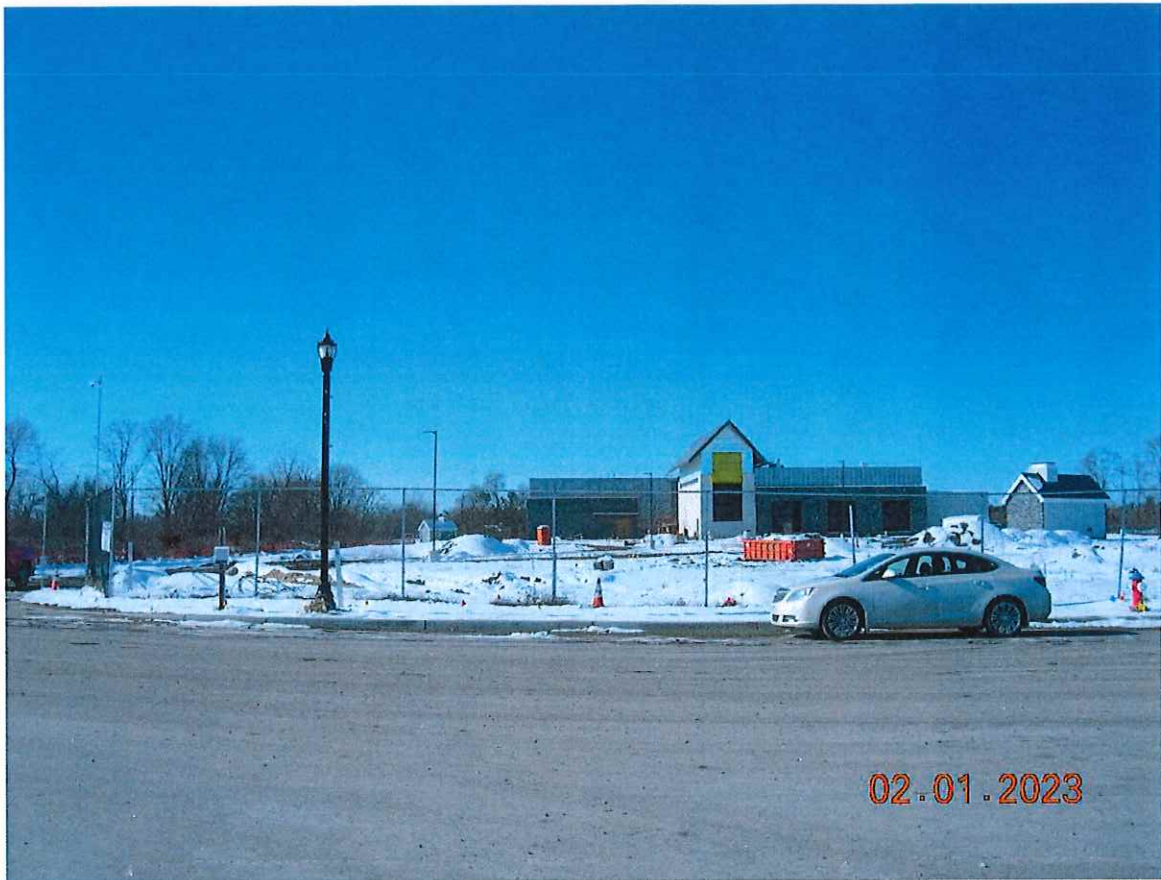
P1. Looking westerly from the current Veterans Parkway terminus / cul-de-sac toward Lot A and the city water production and treatment facility currently under construction.
