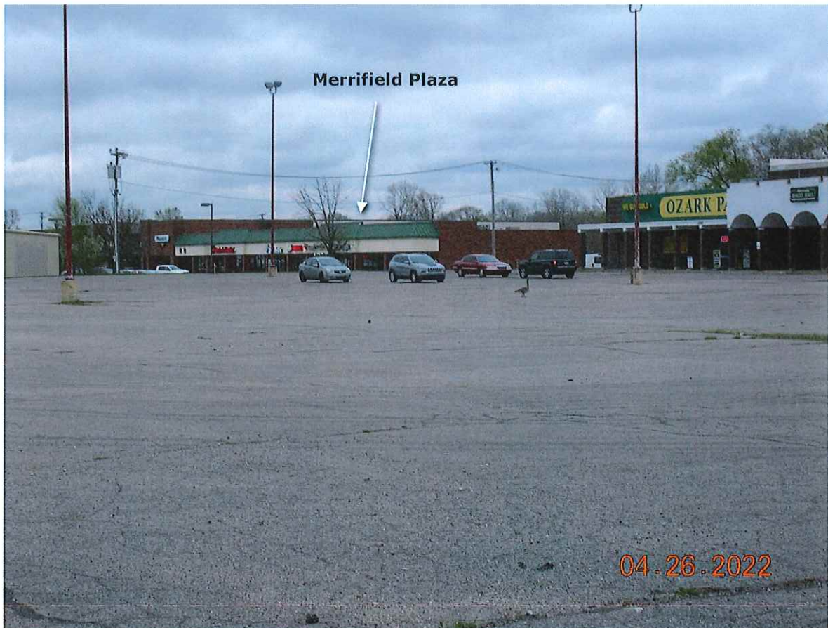
P3. Looking northeasterly from the interior parking area west of the building toward Merrifield Plaza.
