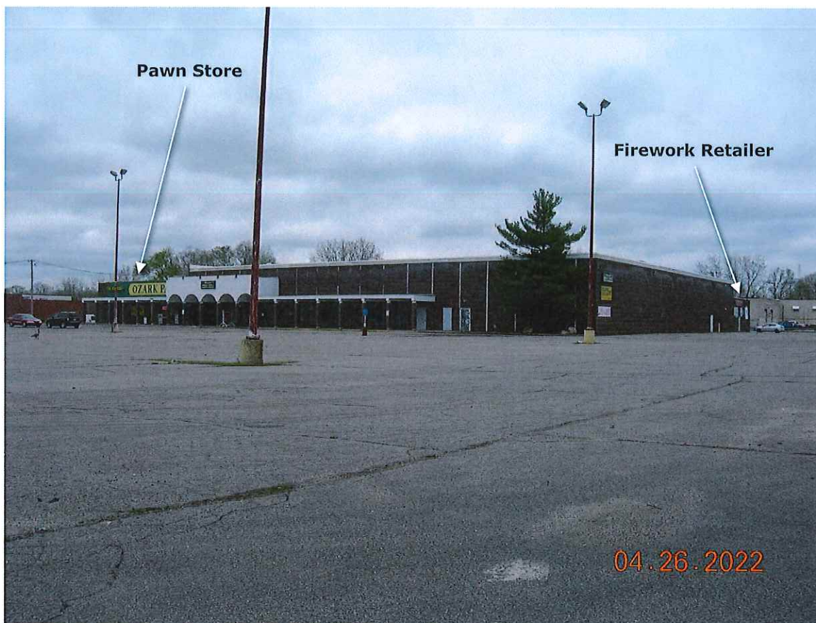
P2. Looking northeasterly from the existing parking lot toward the multi-tenant commercial building.
