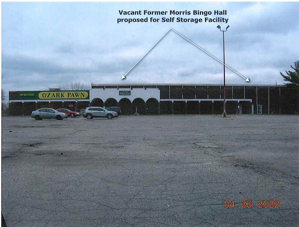
P1. Looking easterly from the parking lot toward the existing multi-tenant commercial building.
