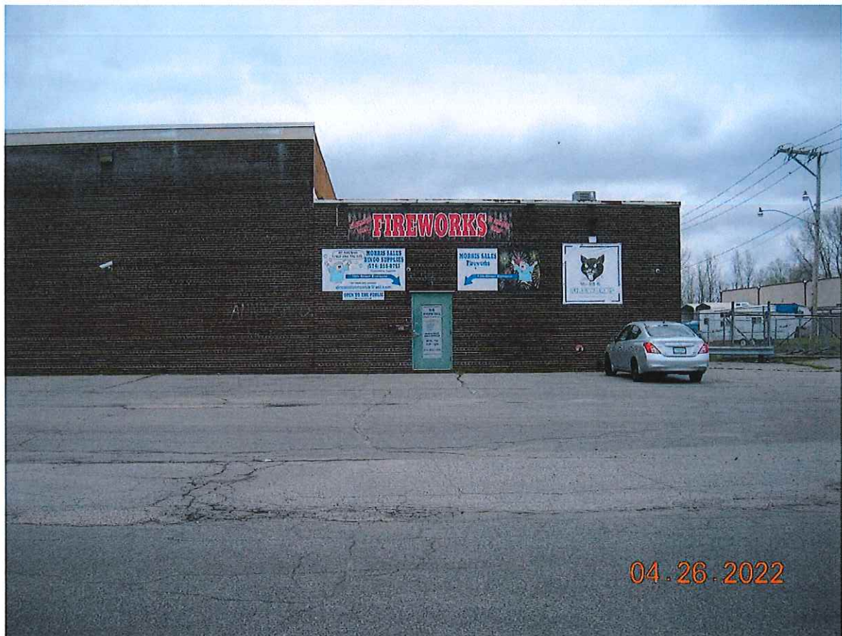
P4. Looking northerly from E. 12 th Street toward Mishawaka Fireworks in the southeast corner of the building.
