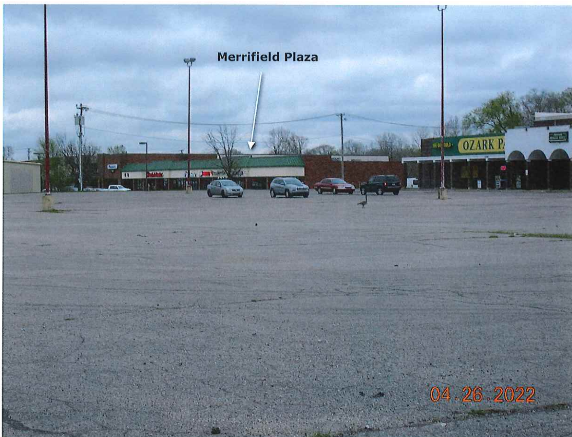
P3. Looking northeasterly from the interior parking area west of the building toward Merrifield Plaza.
