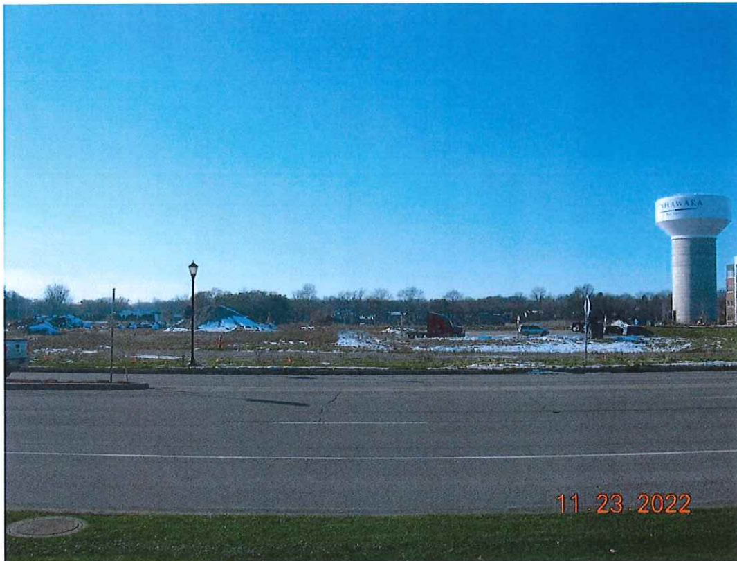
Looking west from Gumwood Road
