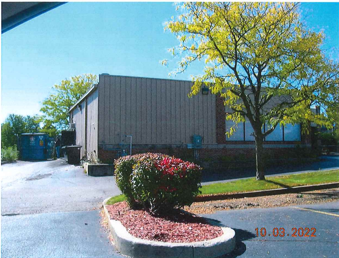
P2. Looking southerly toward the existing building from the property to the north (Arby's).
