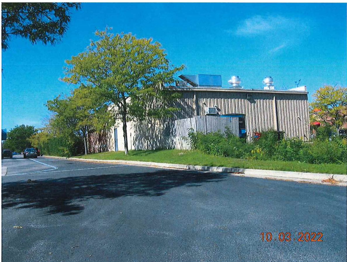
P3. Looking northwesterly toward the rear of the existing building from the property to the south (Culver's).
