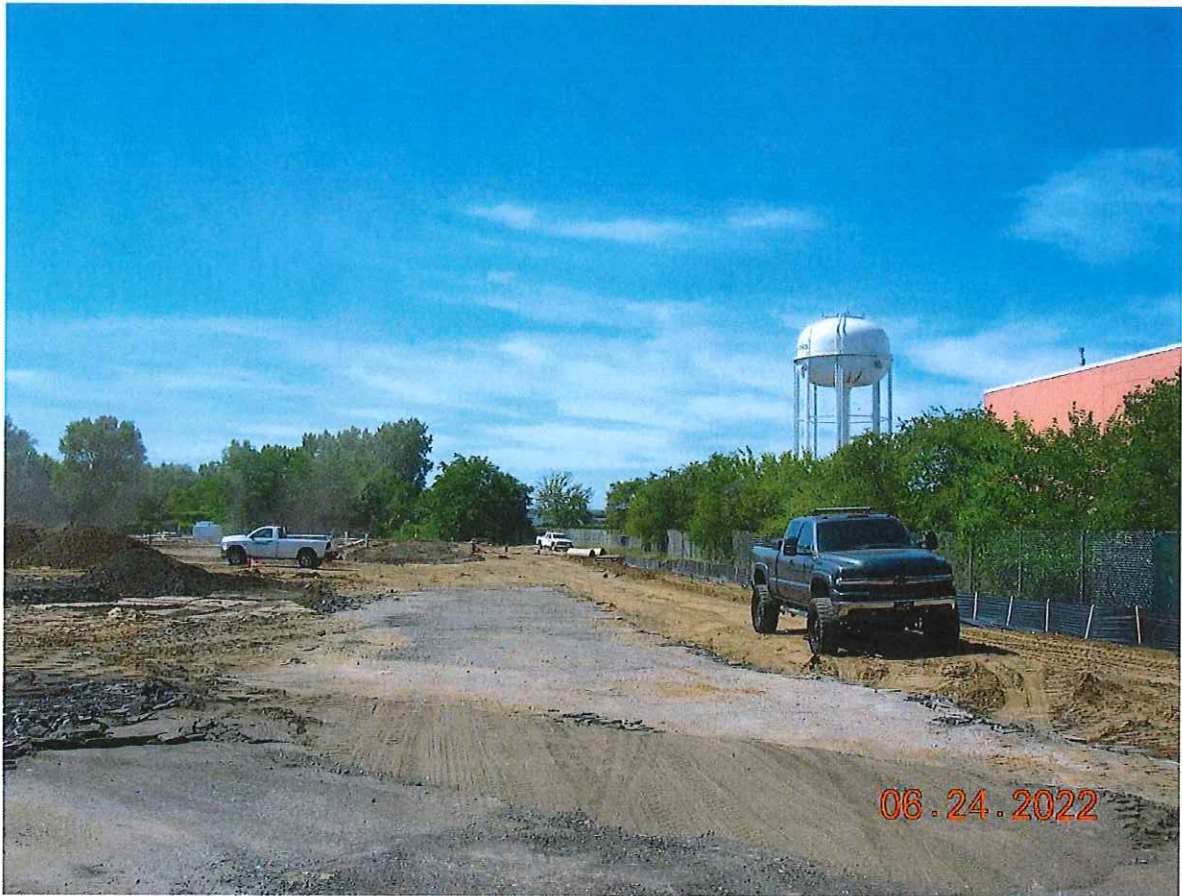
P3. Looking into proposed Lot 2 (Range USA - 655 W. University Dr.) currently under construction from the existing and future access drive.
