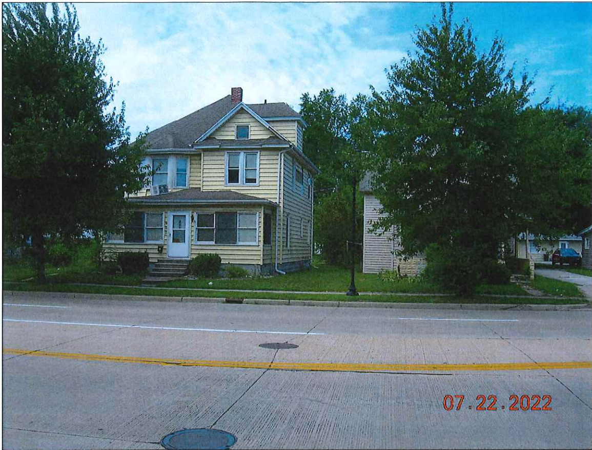
View of home to the south
