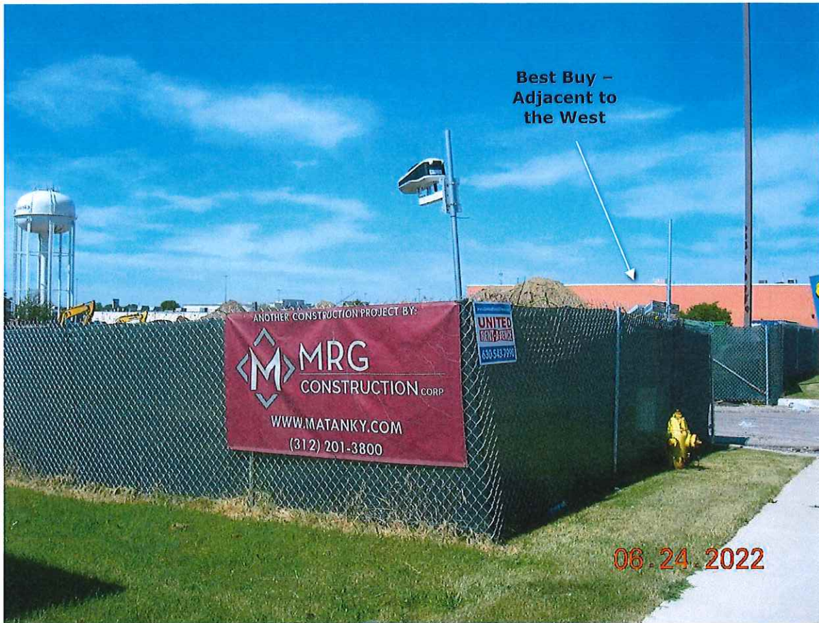
P1. Looking southwesterly from the northeast corner of the property along W. University Drive.
