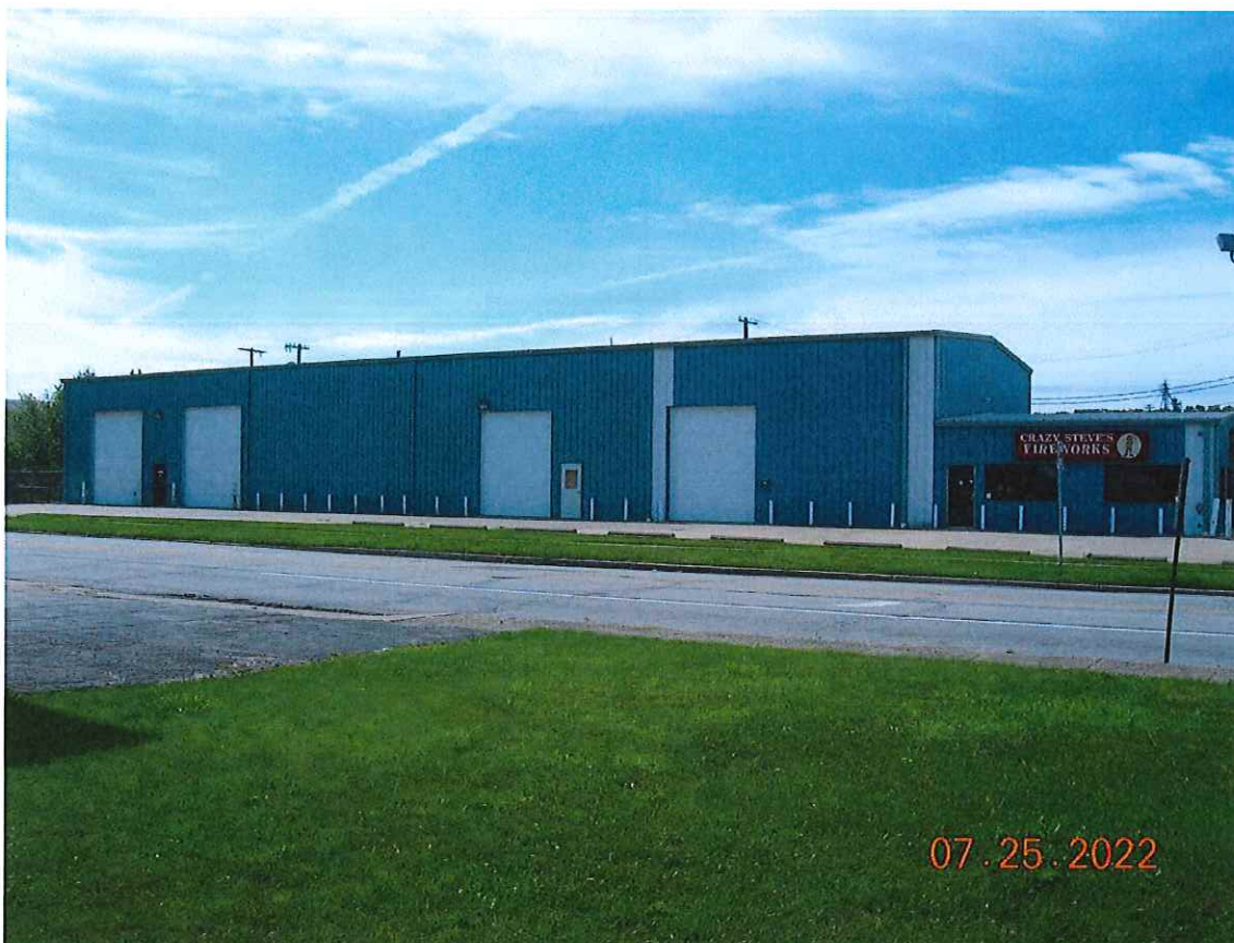
Looking directly south across Eighth Street
