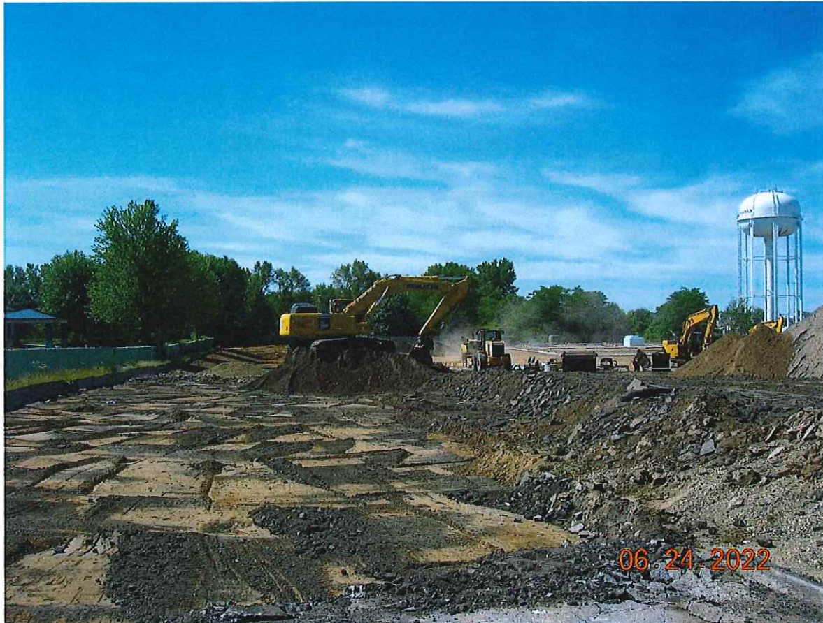
P2. Looking into proposed Lot 1 from the current access point along W. University Drive.
