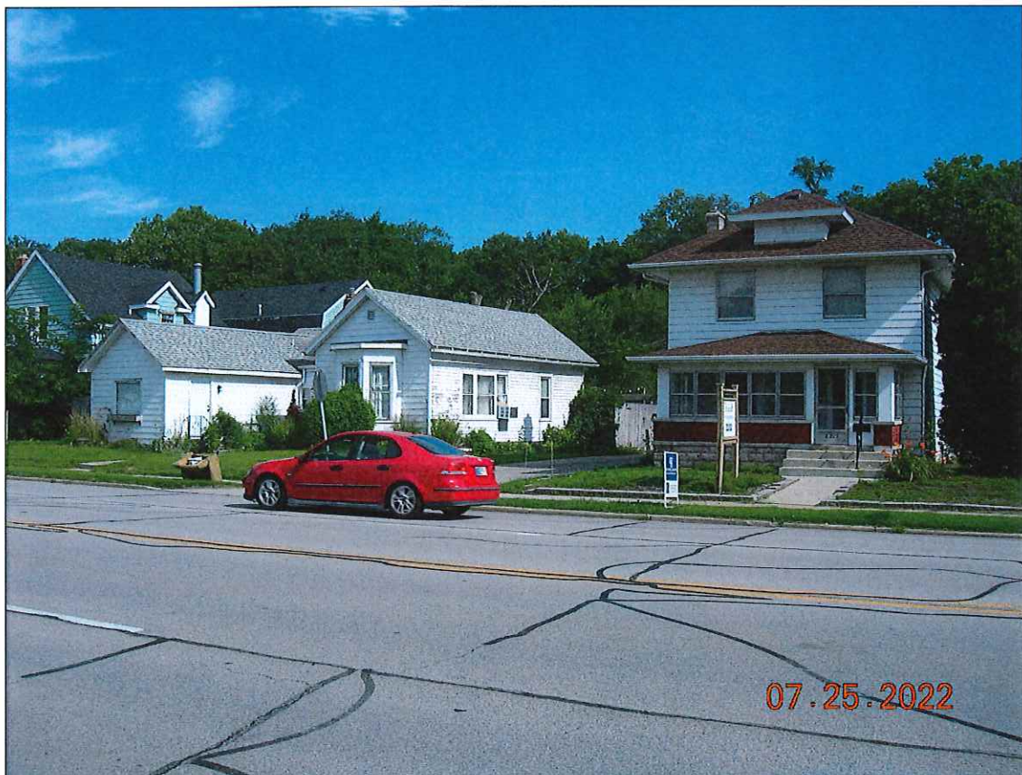
View of residential to the west
