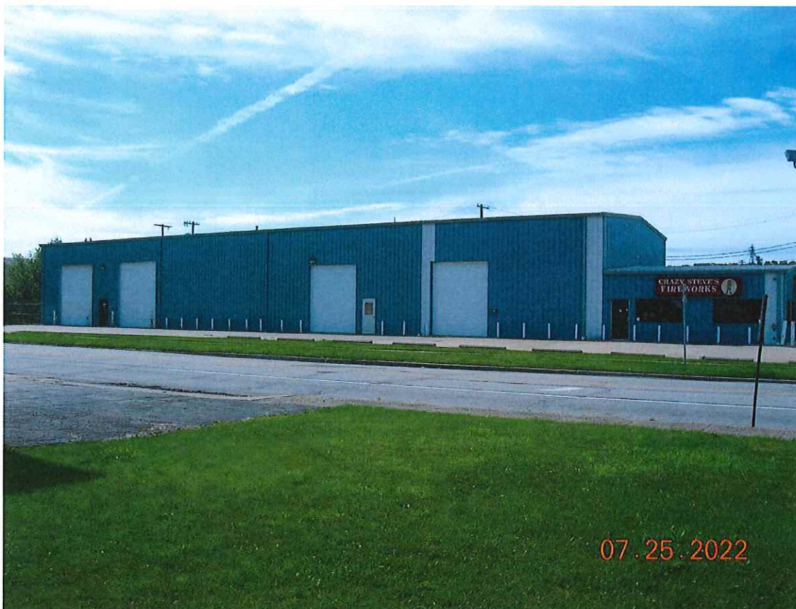
Looking directly south across Eighth Street
