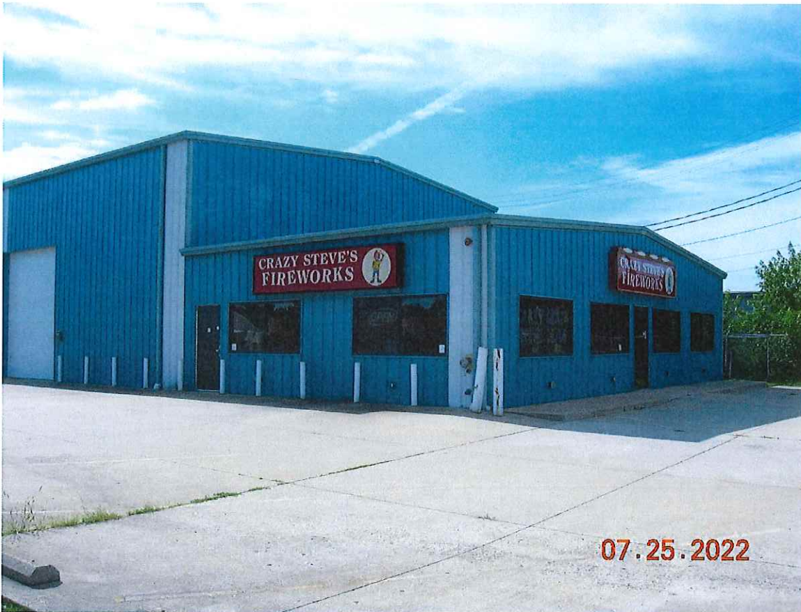
The existing retail area facing Logan Street
