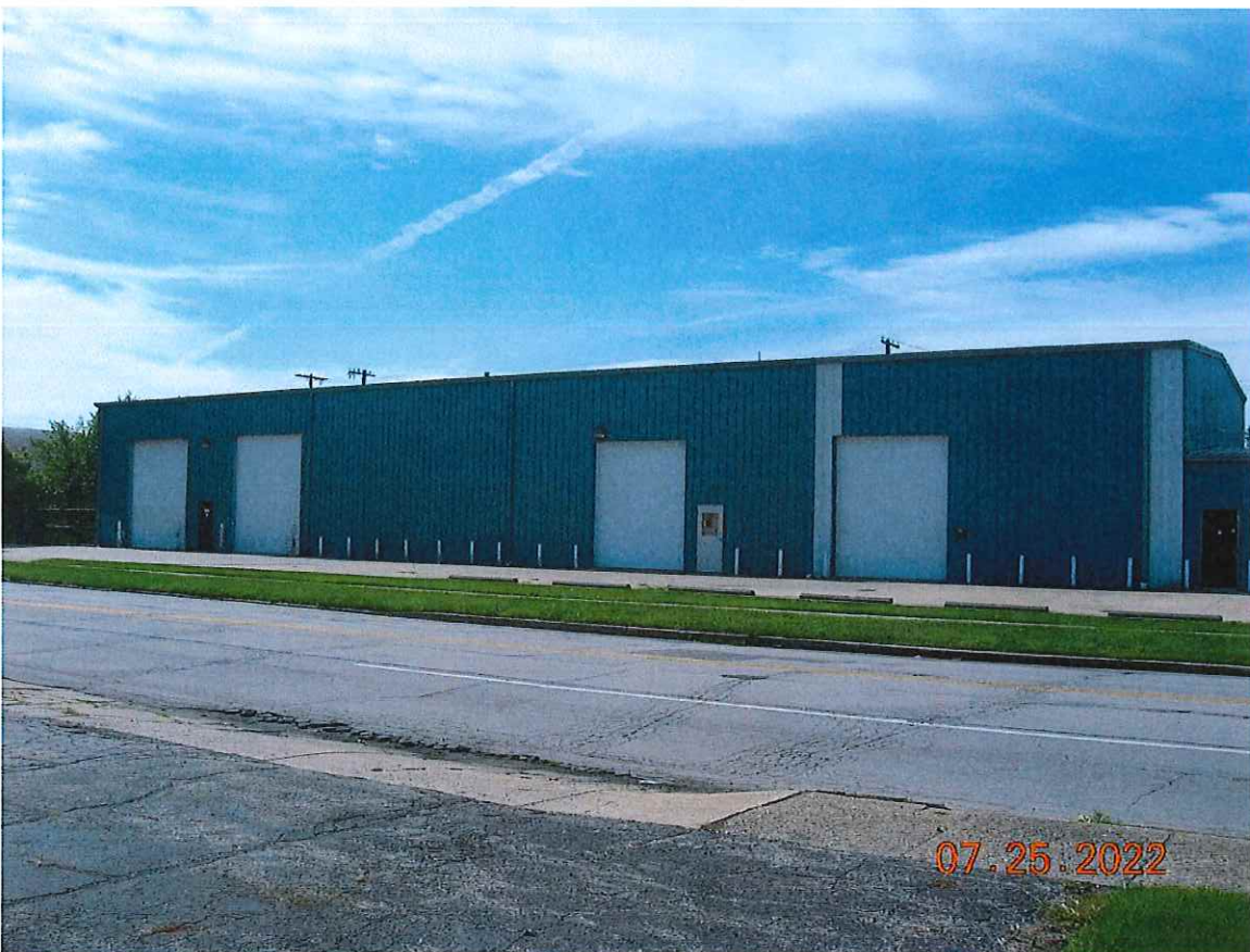
The existing storage facing Eighth Street
