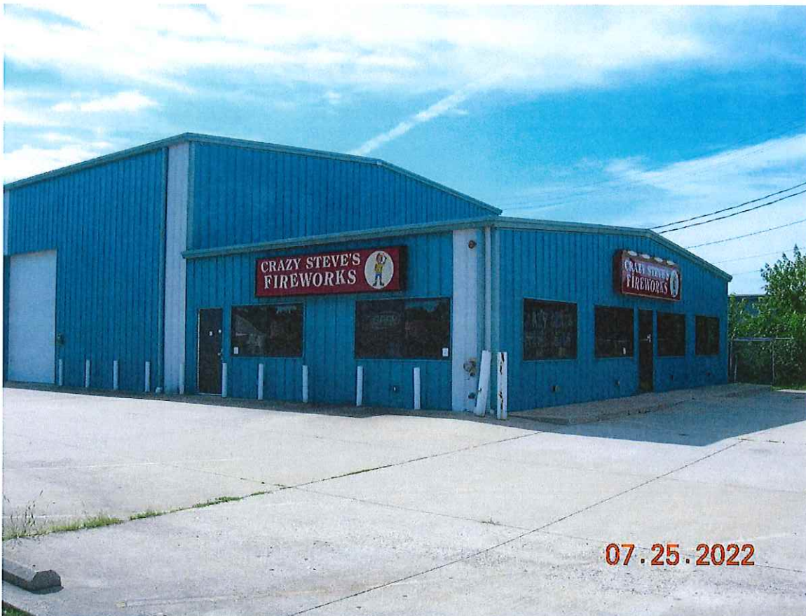
The existing retail area facing Logan Street
