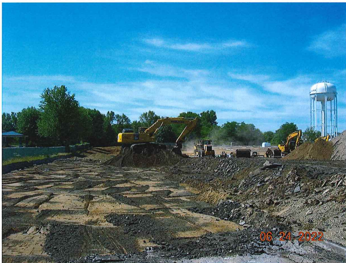
P2. Looking into proposed Lot 1 from the current access point along W. University Drive.
