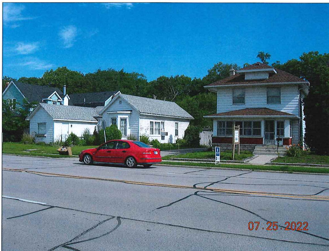
View of residential to the west
