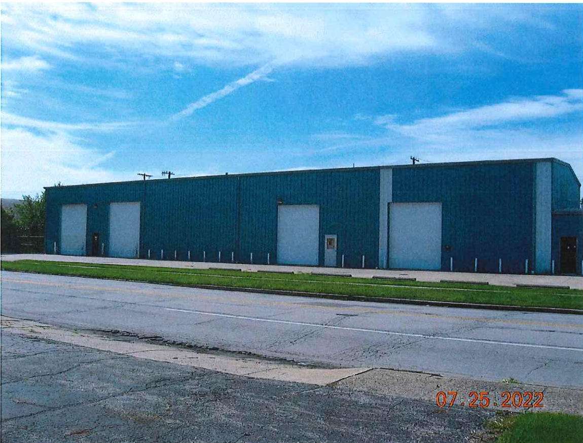
The existing storage facing Eighth Street
