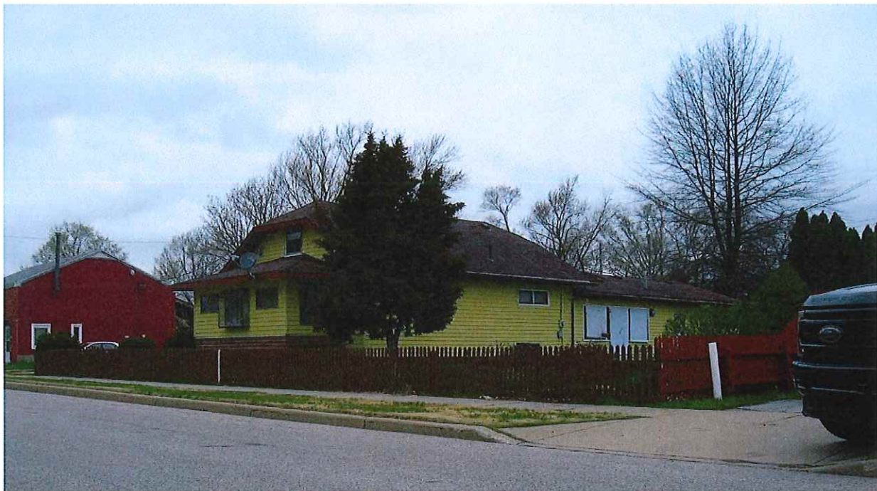
A view of the house to the west
