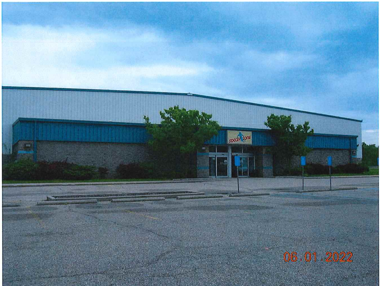
Front view (west elevation)
