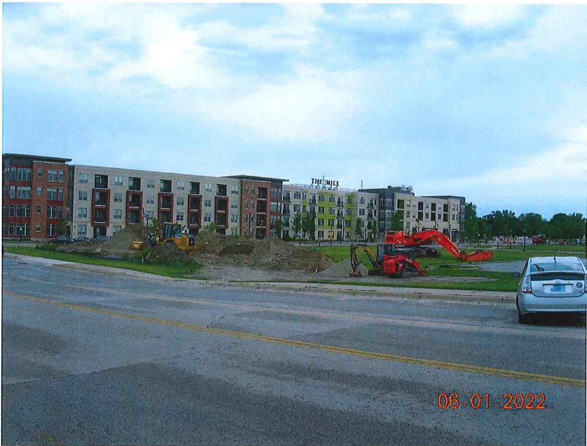
P3. Looking northeasterly toward Parcel 3 from N. Hill St.
