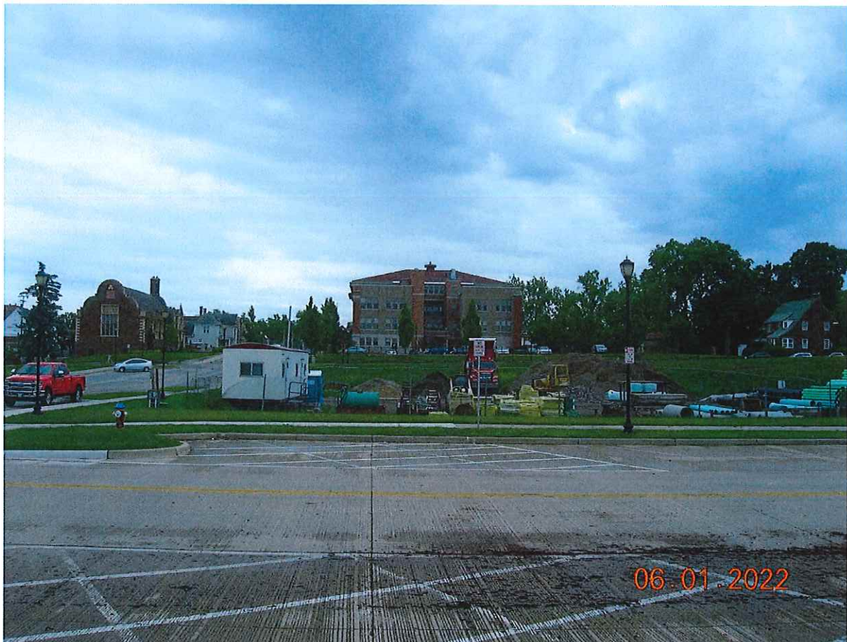
P4. Looking southerly toward Parcel 1 staging area from W. Front St.
