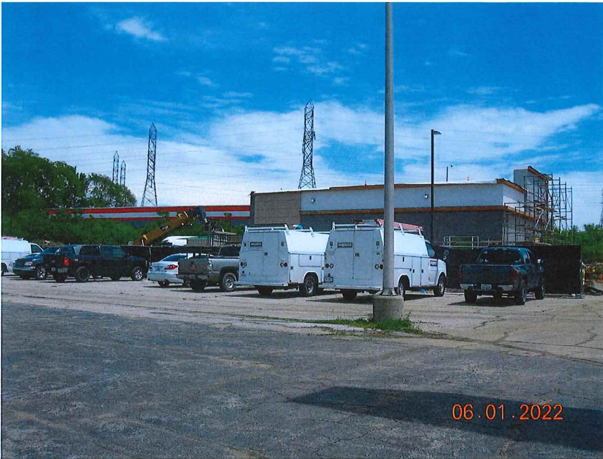
P3. Looking easterly from the parking area between Mishawaka Inn and Dunkin' Donuts under construction.
