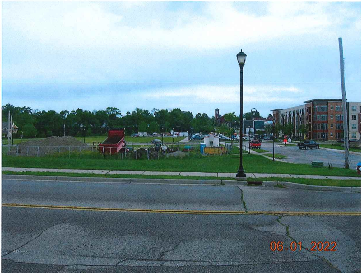
P2. Looking northerly toward Parcel 2 and Parcel 1 staging area to the north from W. First St.
