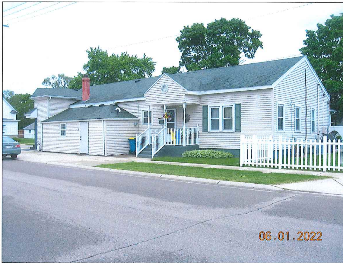
View of rear living area from Cleveland Street
