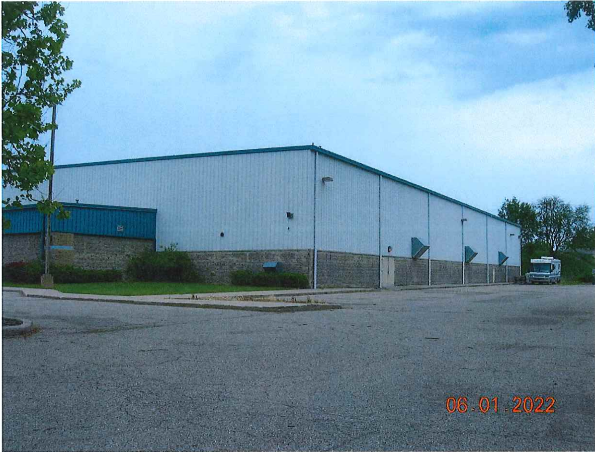
Side facing Toll Road (south elevation)
