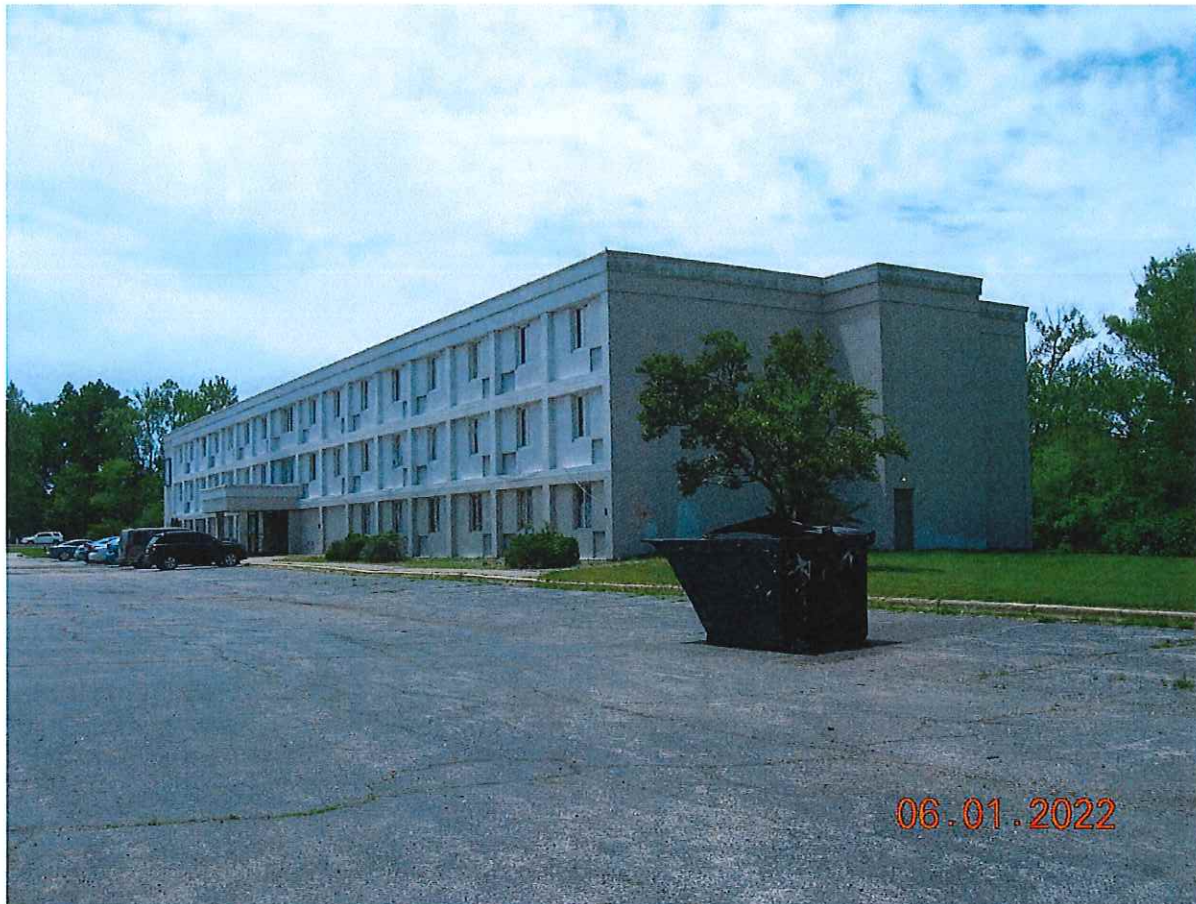
P4. Looking southwest toward the existing Mishawaka Inn from the general location of the proposed new building.
