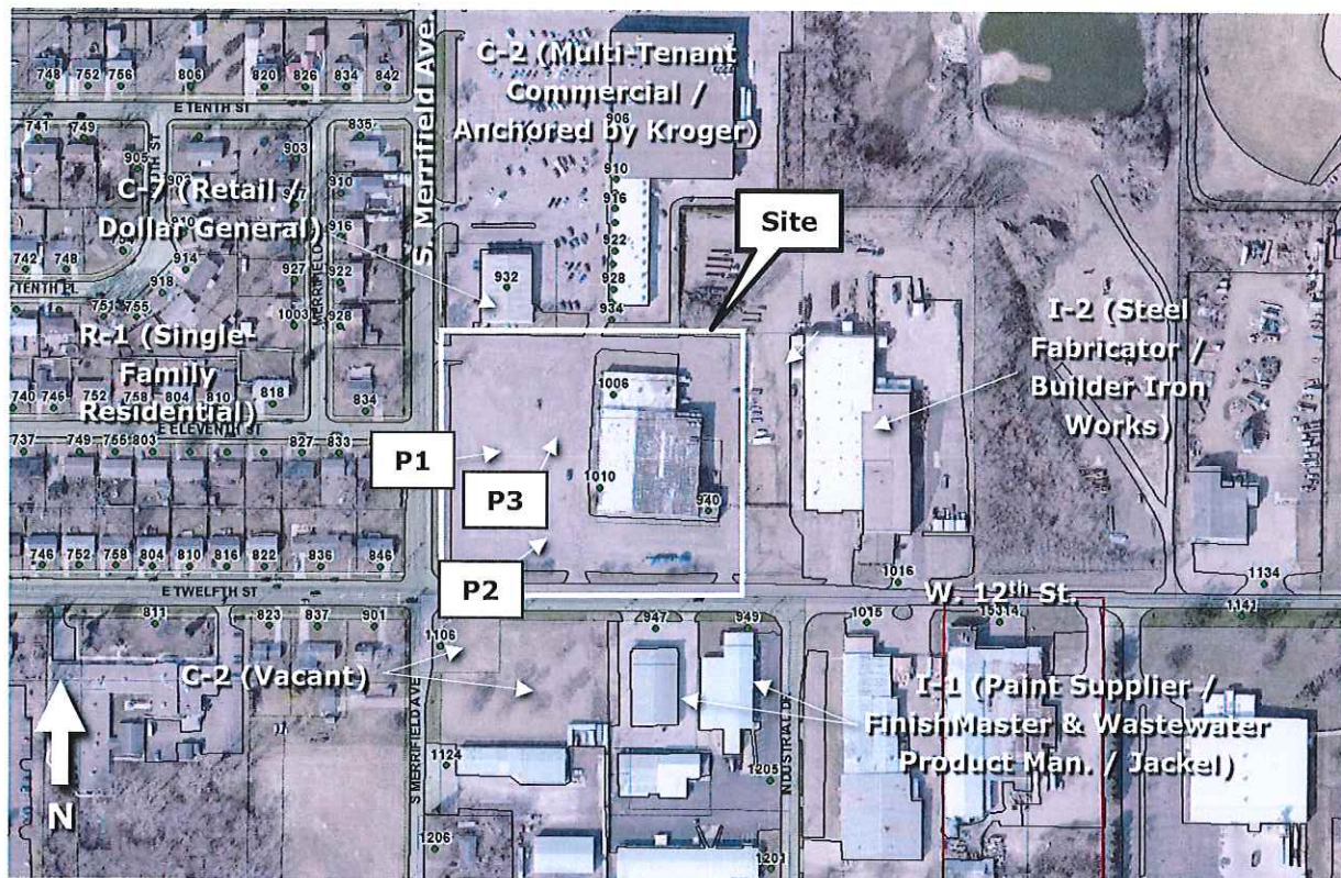
Aerial Photograph Existing Multi-Tenant Commercial Building Proposed for Reuse as Indoor Storage 1010 S. Merrifield Ave.
