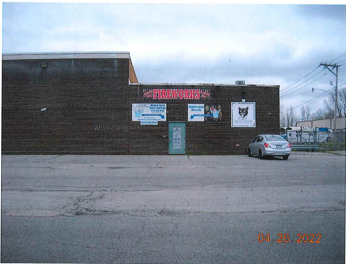
P4. Looking northerly from E. 12 th Street toward Mishawaka Fireworks in the southeast corner of the building.
