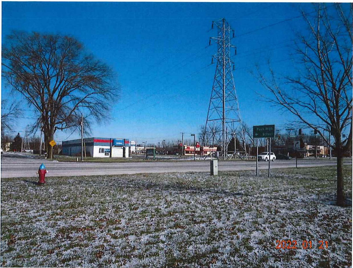
P7. Looking northeasterly from LWE toward the existing carwash facility at 4506 LWE to be razed.
