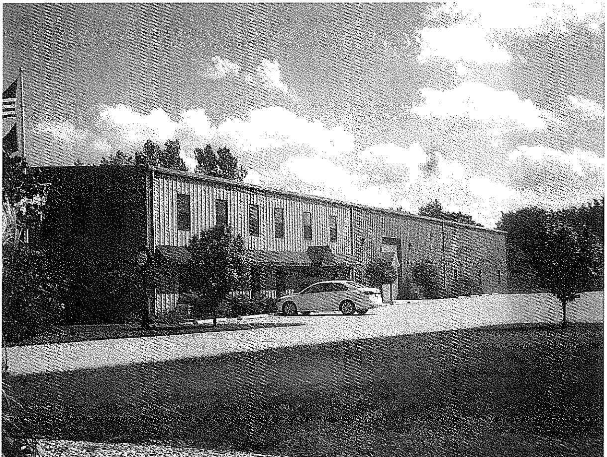
Views looking onto existing building
