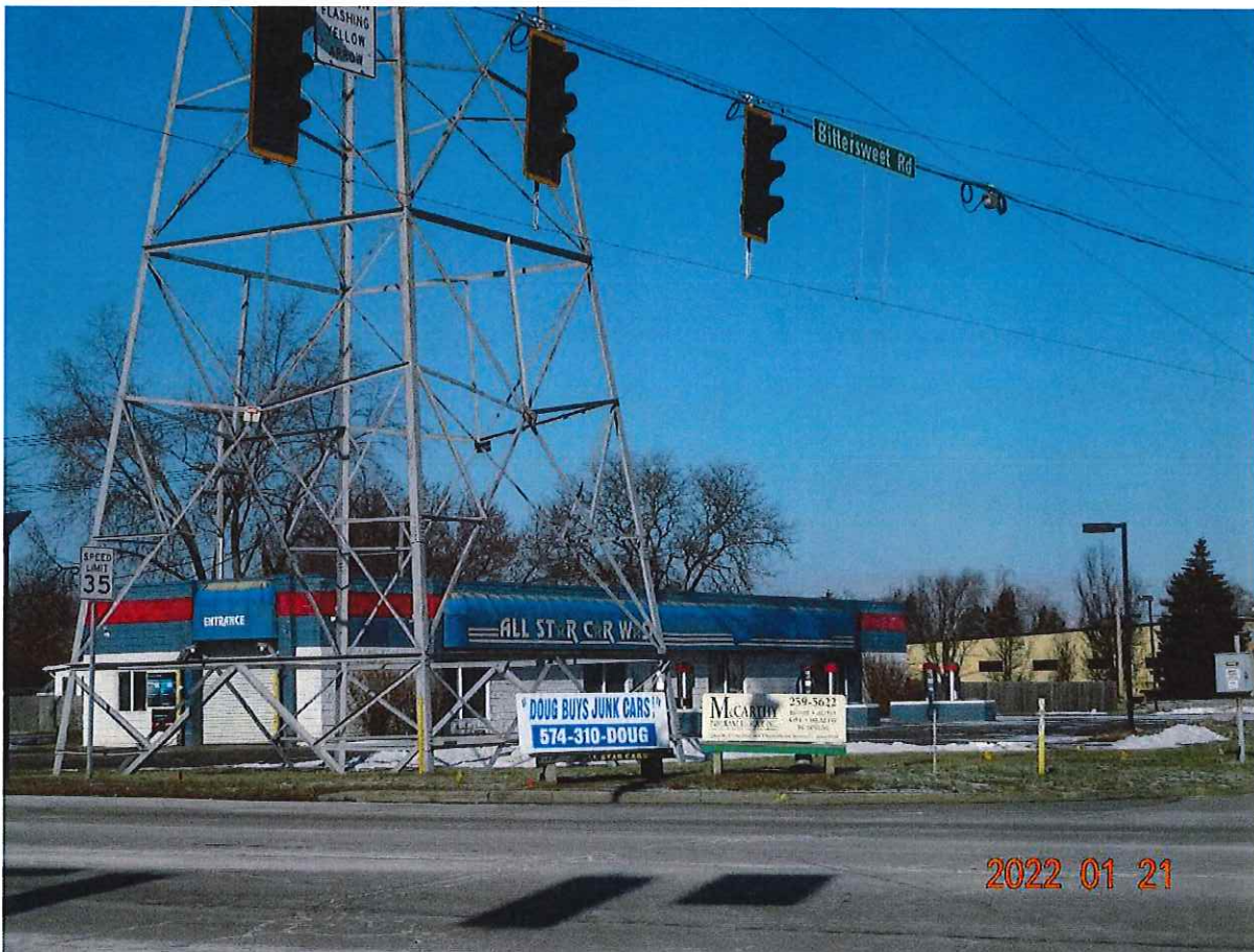
P6. Looking northwesterly from LWE toward the existing carwash facility at 4506 to be razed.
