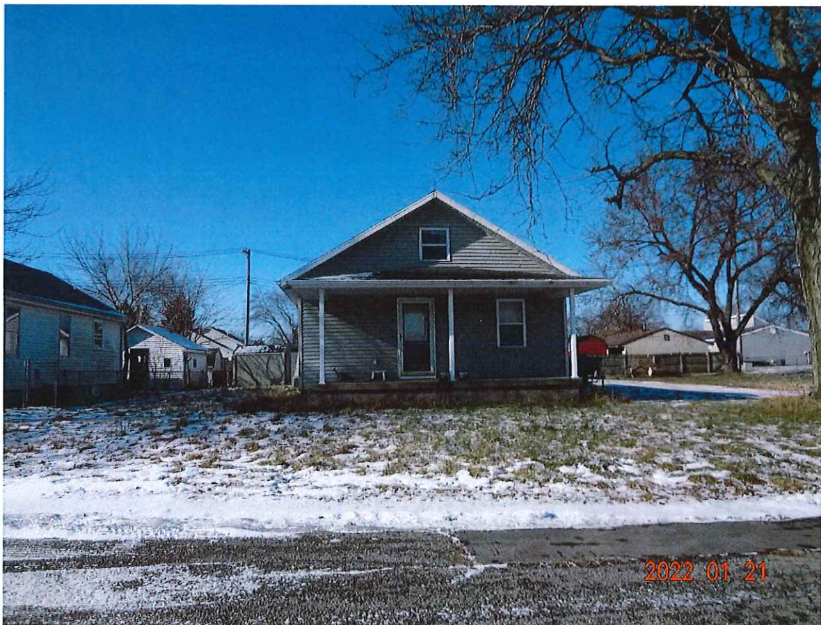
P2. Looking westerly toward 123 Wayne Street, one of three parcels to be rezoned and the buildings razed.
