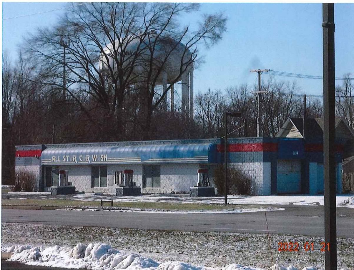
P5. Looking southwesterly from Bittersweet Rd. toward the existing carwash facility at 4506 LWE to be razed.
