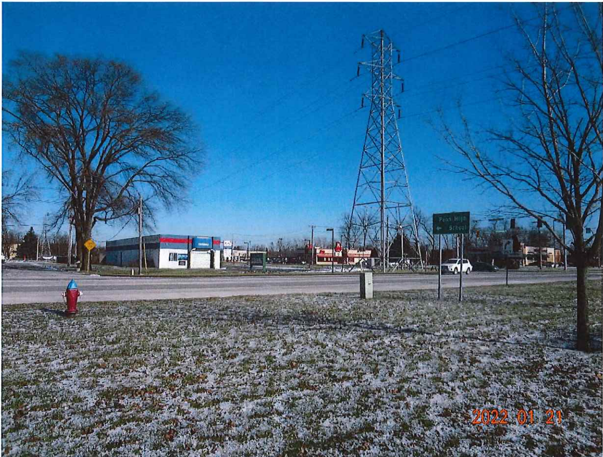
P7. Looking northeasterly from LWE toward the existing carwash facility at 4506 LWE to be razed.
