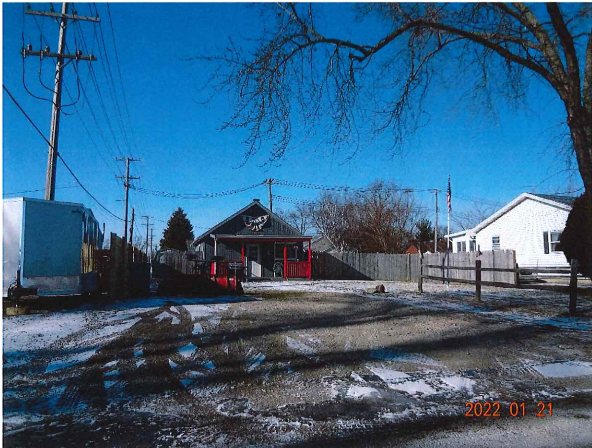
P4. Looking westerly toward 107 Wayne Street, one of three parcels to be rezoned and the buildings razed.
