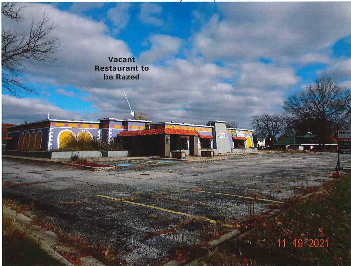
P1. Looking northeasterly toward the existing restaurant from the Cleveland Rd. (S.R. 23) access.
