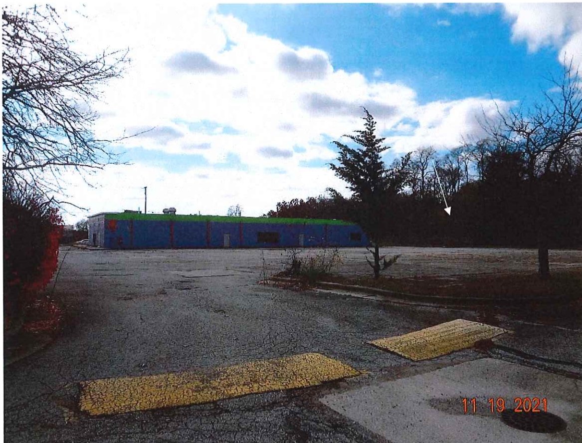
P5. Looking southwesterly toward the property from the adjacent access drive to the north.
