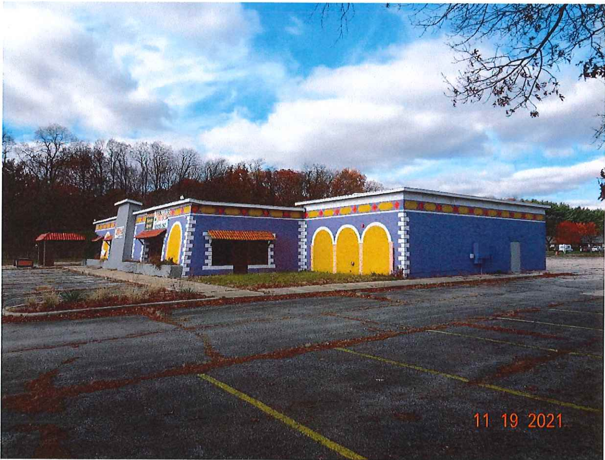
P6. Looking northwesterly toward of the existing building from the east.
