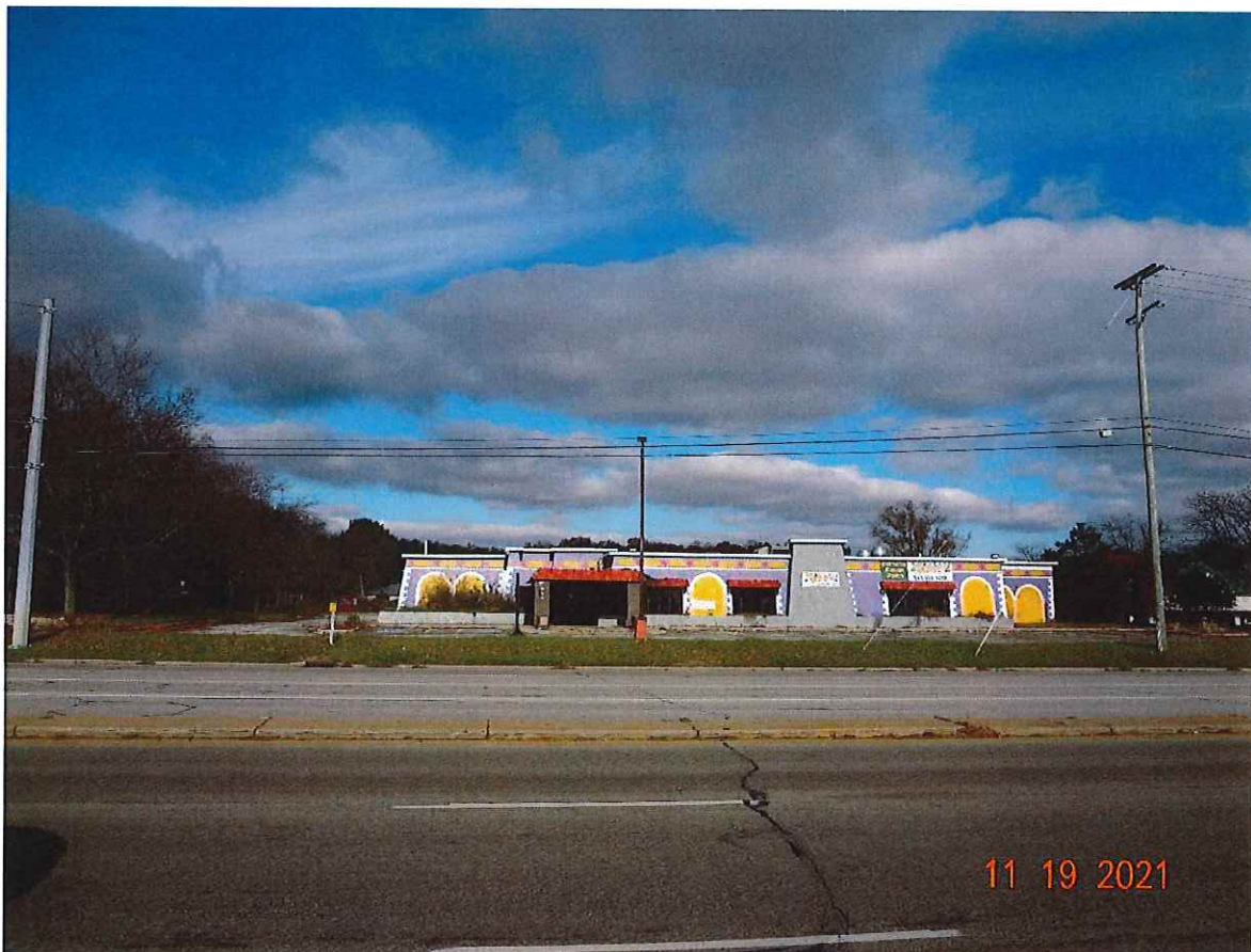
P7. Looking northerly toward the property and existing building from south of S.R. 23.
