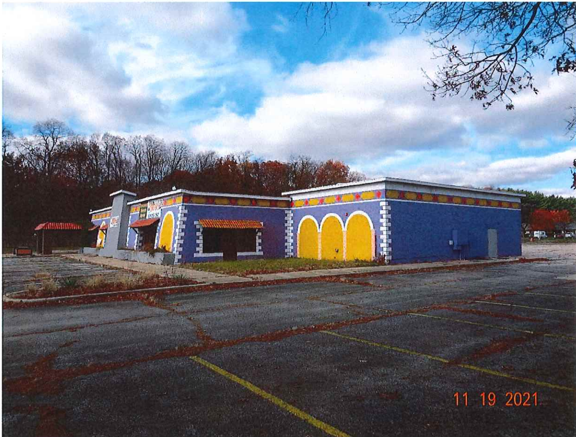
P6. Looking northwesterly toward of the existing building from the east.
