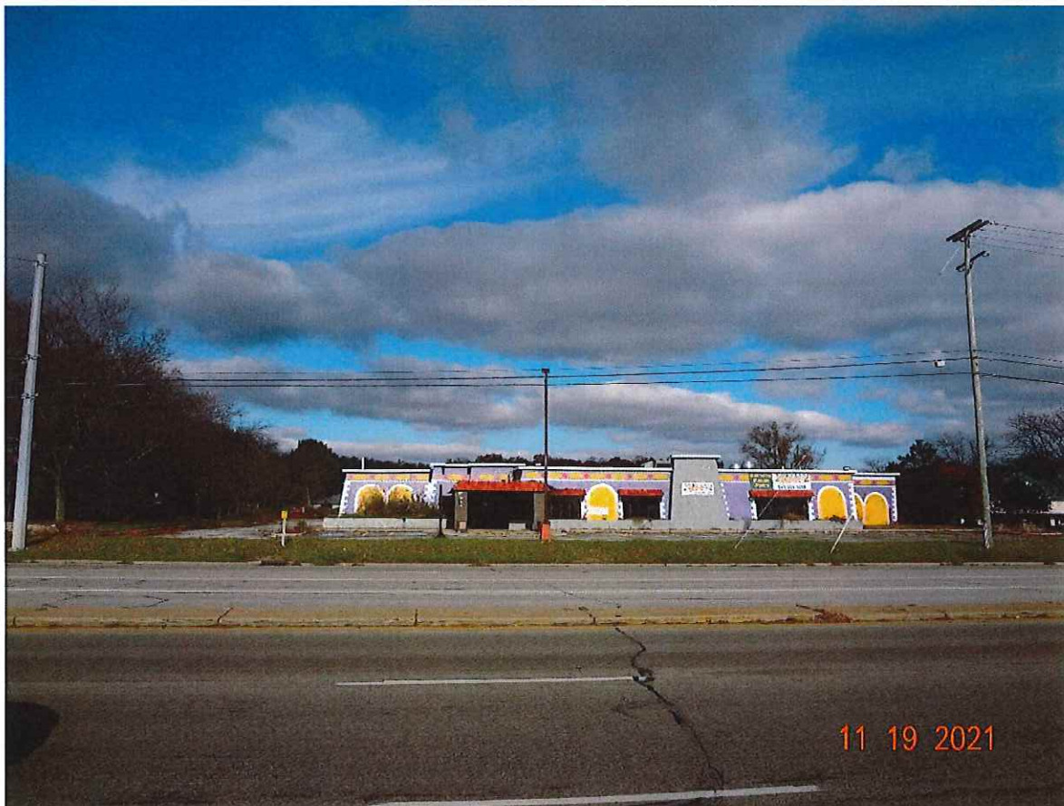
P7. Looking northerly toward the property and existing building from south of S.R. 23.
