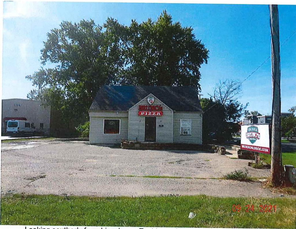
Looking southerly from Lincolnway East toward Bruno's Pizza (12452 LWE). Front part of parcel is proposed to be zoned C-1 General Commercial with no change in use.
