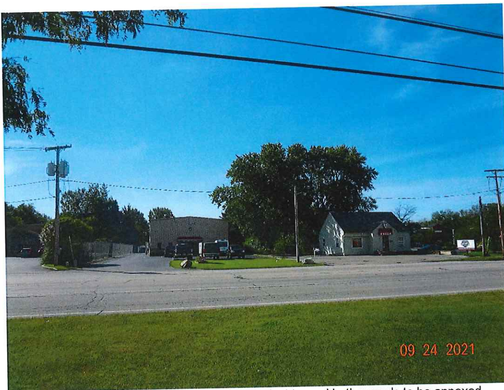
Looking southerly from north of Lincolnway East toward both parcels to be annexed. .
