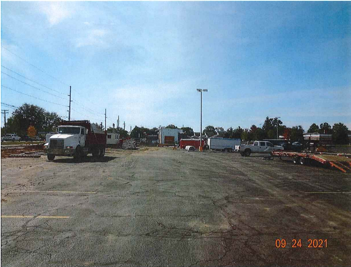
A view of the site from the northern part of the parking lot
