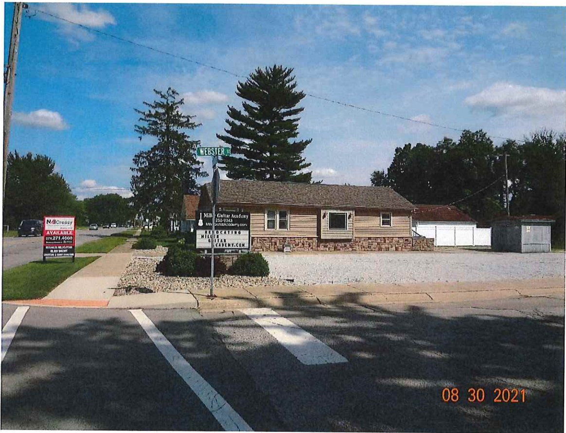
A view of the building and sign from Webster
