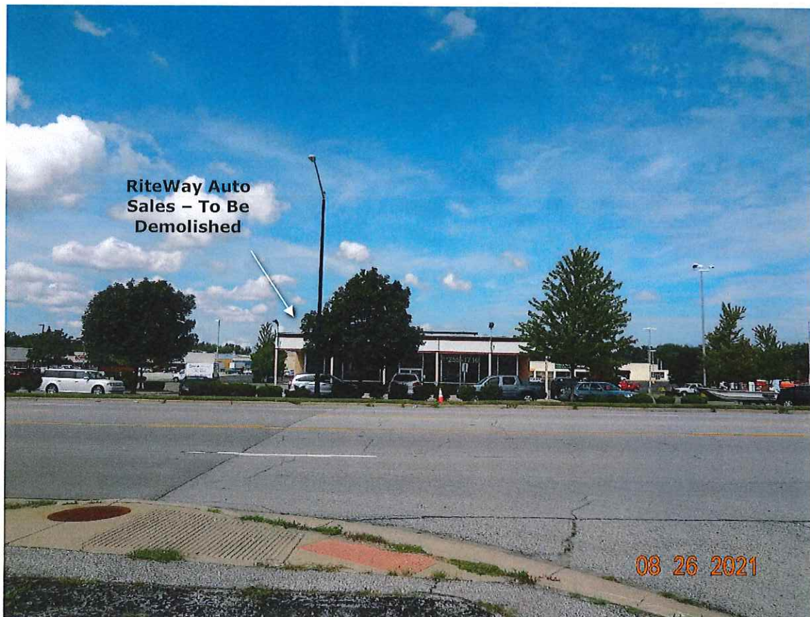
P7. Looking northerly from south of W. McKinley Avenue toward the property to be rezoned.
