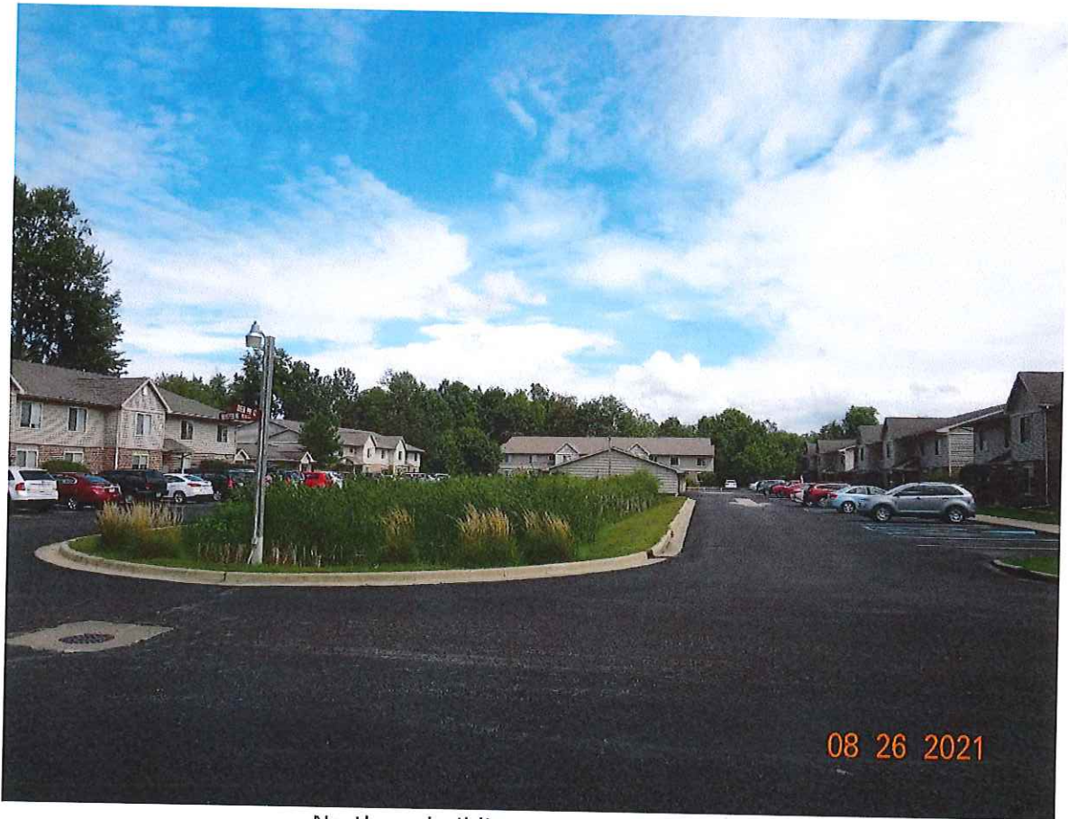
Northern buildings on Green Pine Ct
