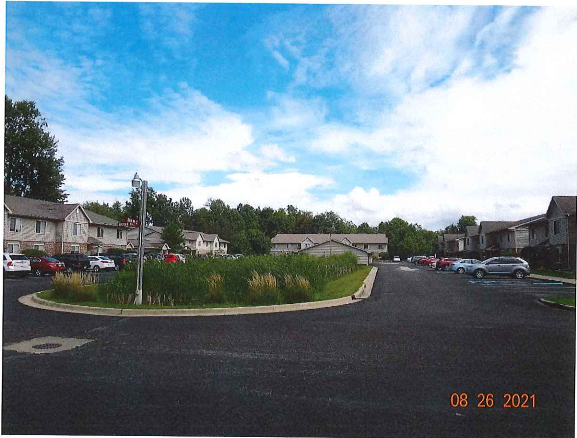
Northern buildings on Green Pine Ct
