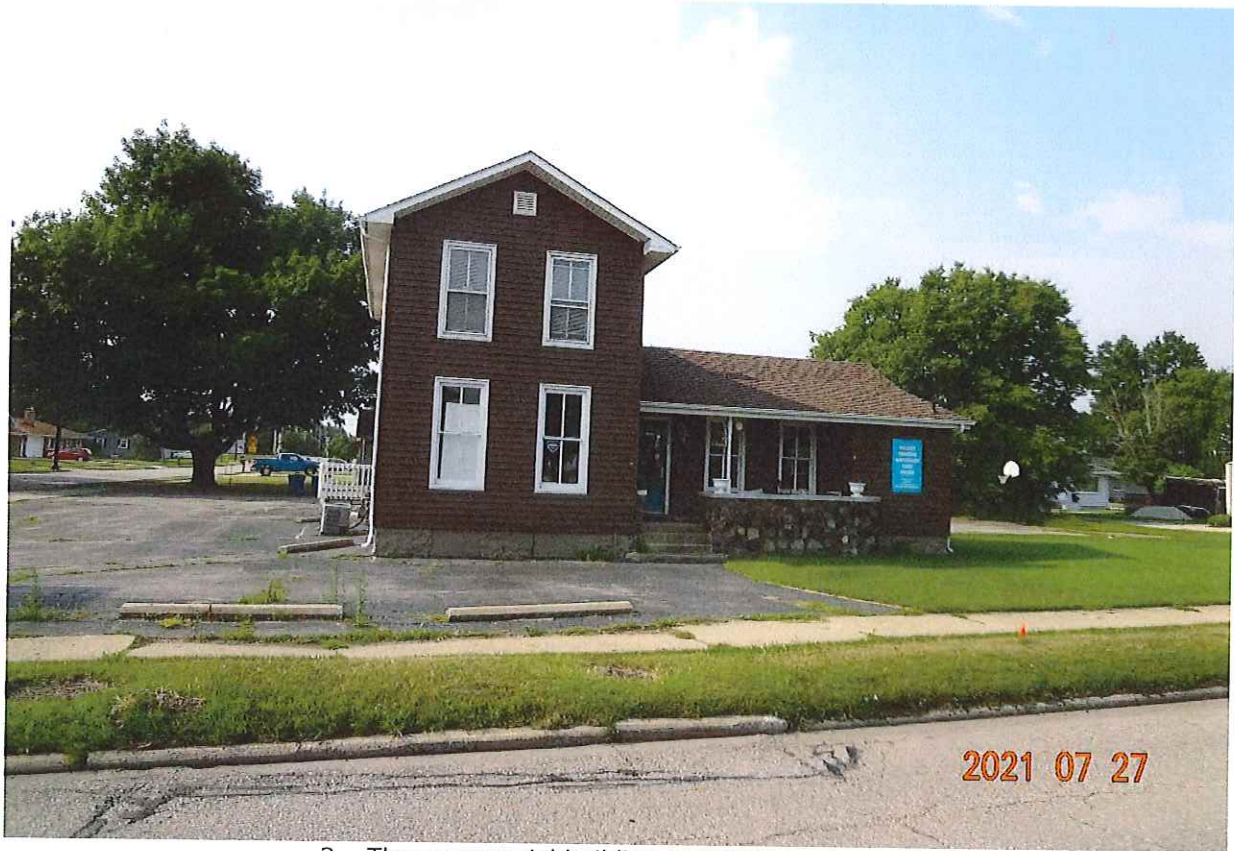
2. The commercial building at 3019 Lincolnway East
