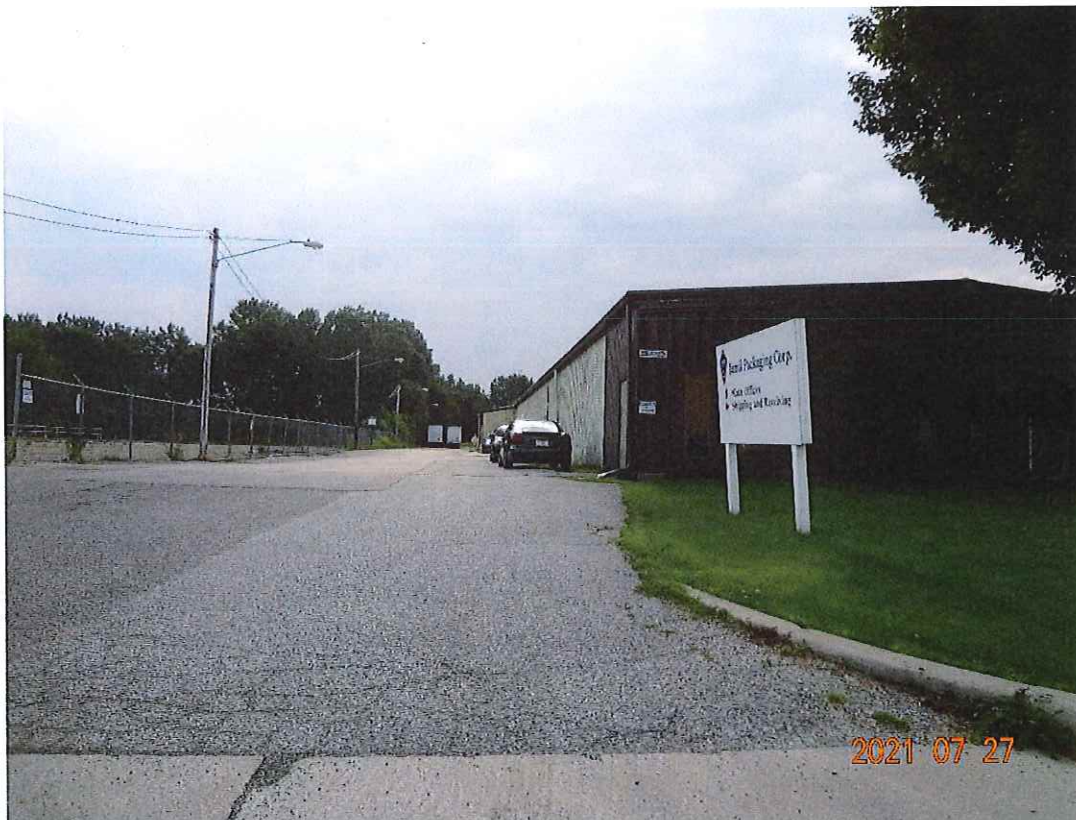
A view towards the rear of the existing business along Industrial Drive
