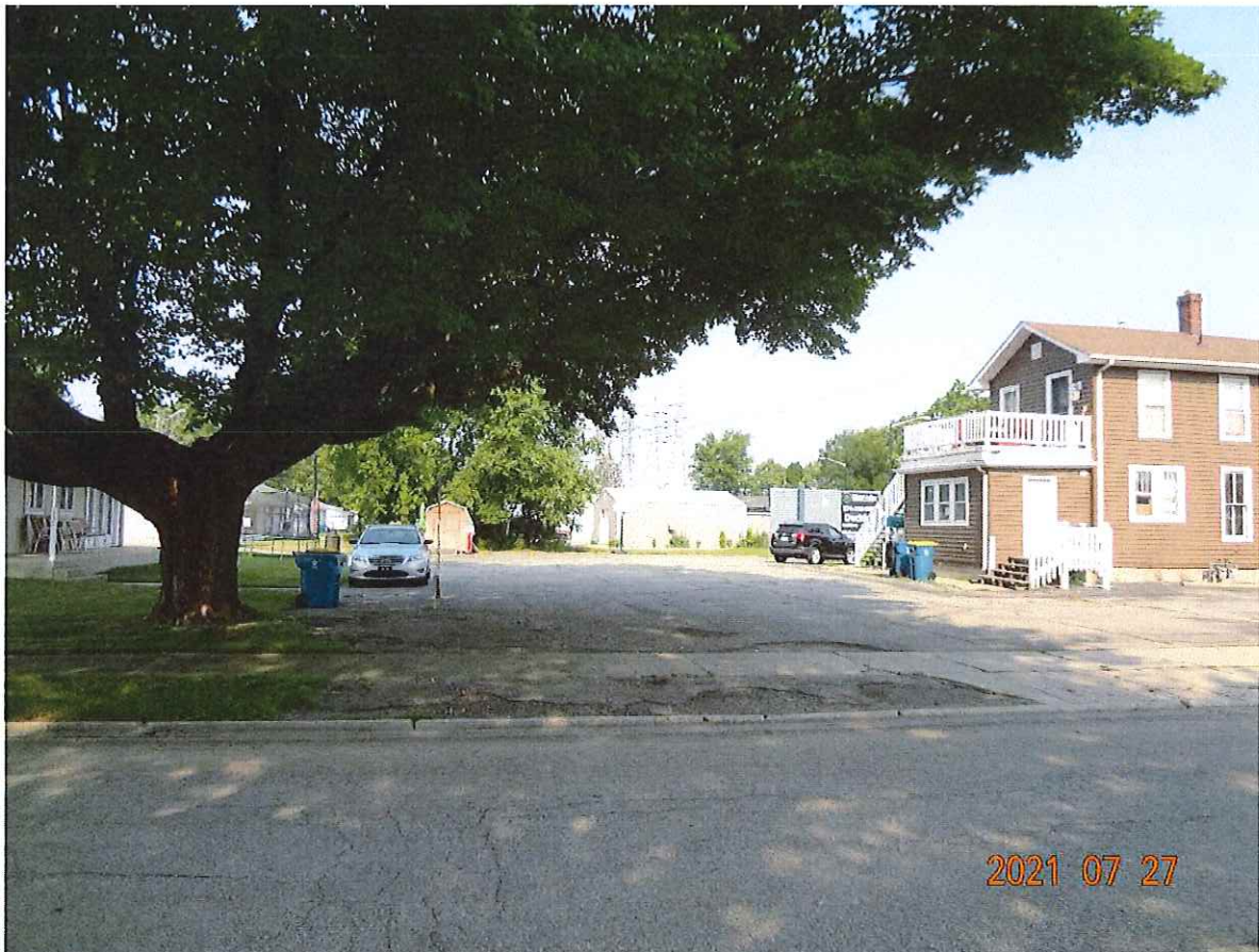
3. Shared access and parking area between the two buildings
