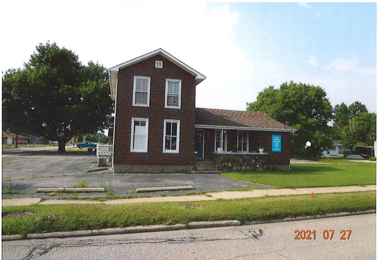
2. The commercial building at 3019 Lincolnway East
