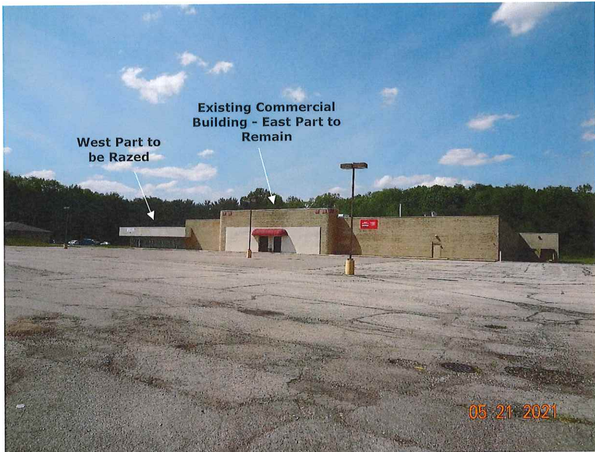
P1. Looking northwesterly toward the existing building from the Grape Road access.
