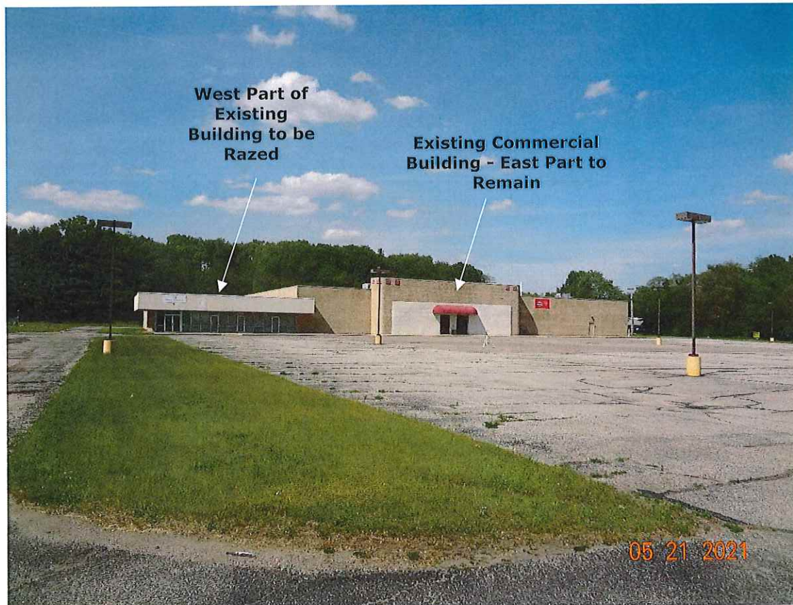
P4. Looking northeasterly toward the existing building from south of the only existing landscape island.
