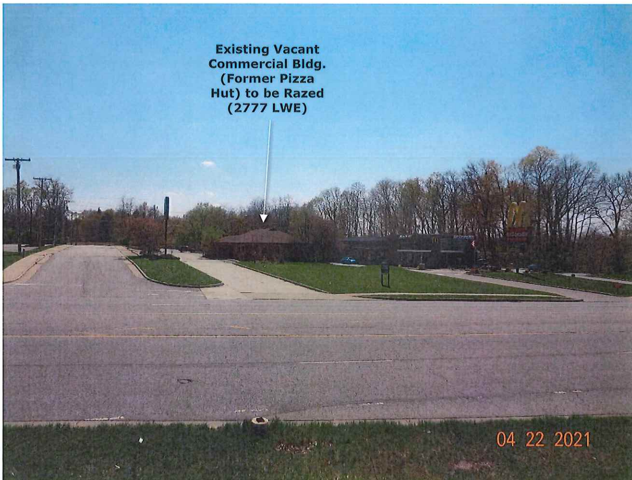
P1. Looking southerly toward the site from north of Lincoln Way East.
