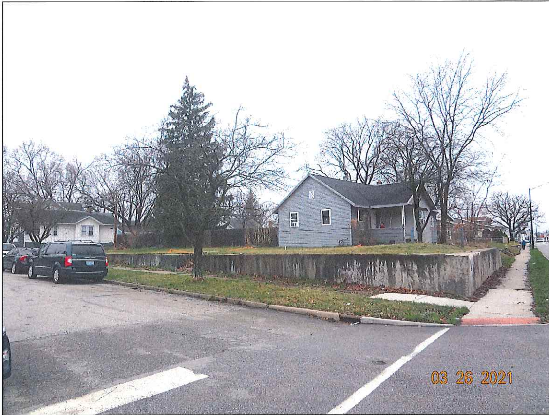
View looking west at the vacant lot
