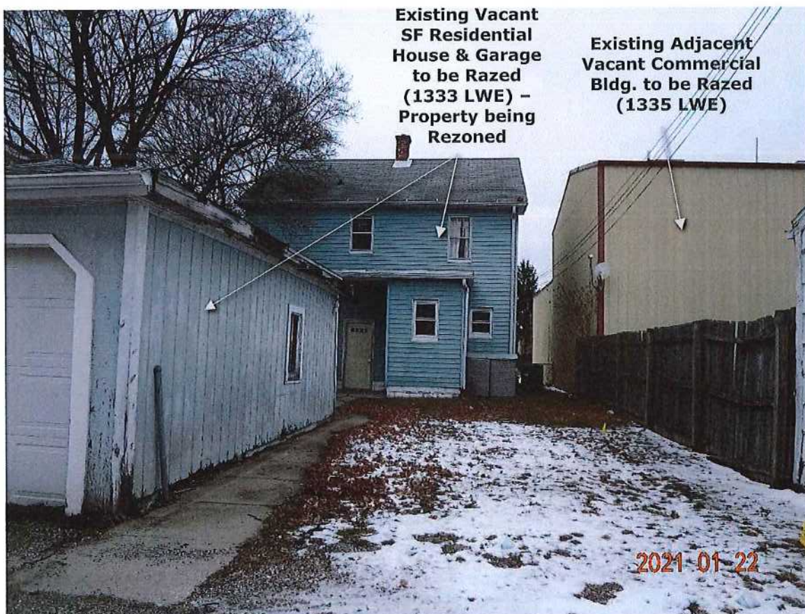
P3. Looking northerly toward the existing house and detached garage from the alley to the south.
