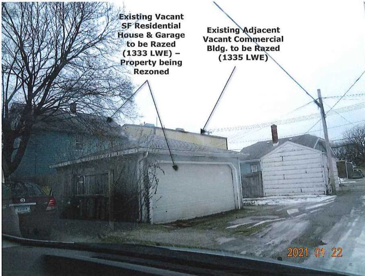
P2. Looking northeasterly toward the existing house and detached garage from the alley to the south.
