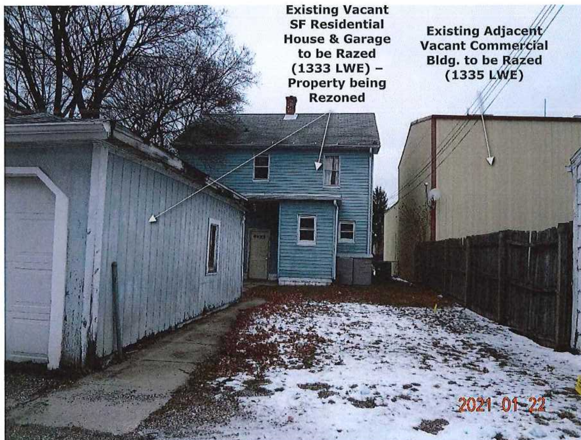
P3. Looking northerly toward the existing house and detached garage from the alley to the south.
