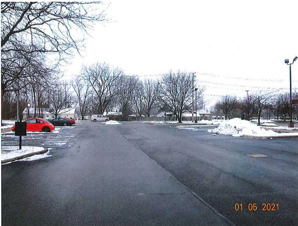
P2. Looking westerly along the existing access drive (Honeysuckle Ln) to the south.
