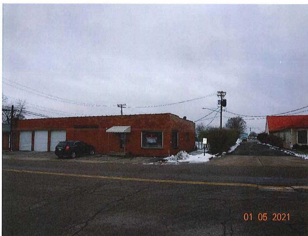
Front view of 411 S Main
