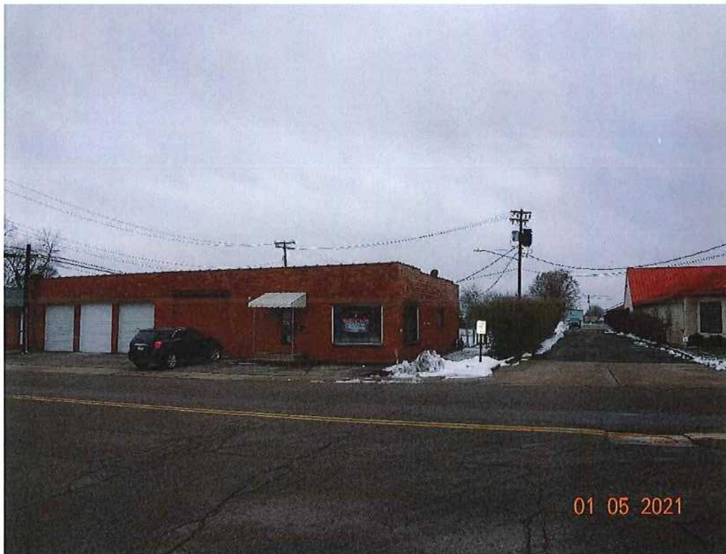
Front view of 411 S Main
