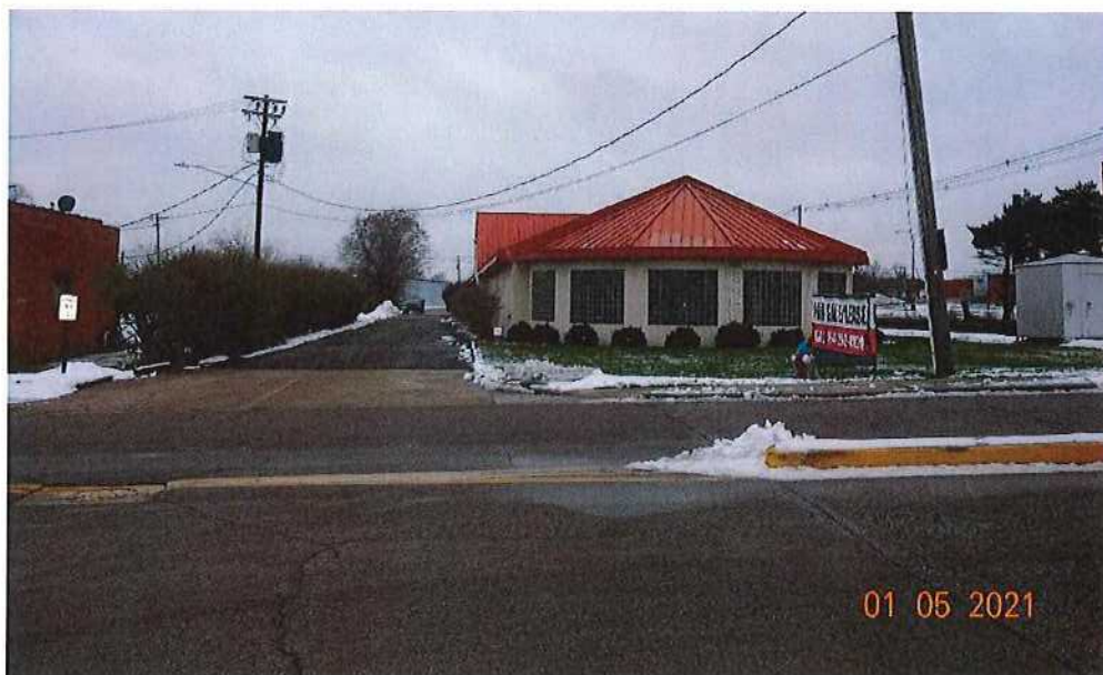
Front view of 403 S Main
