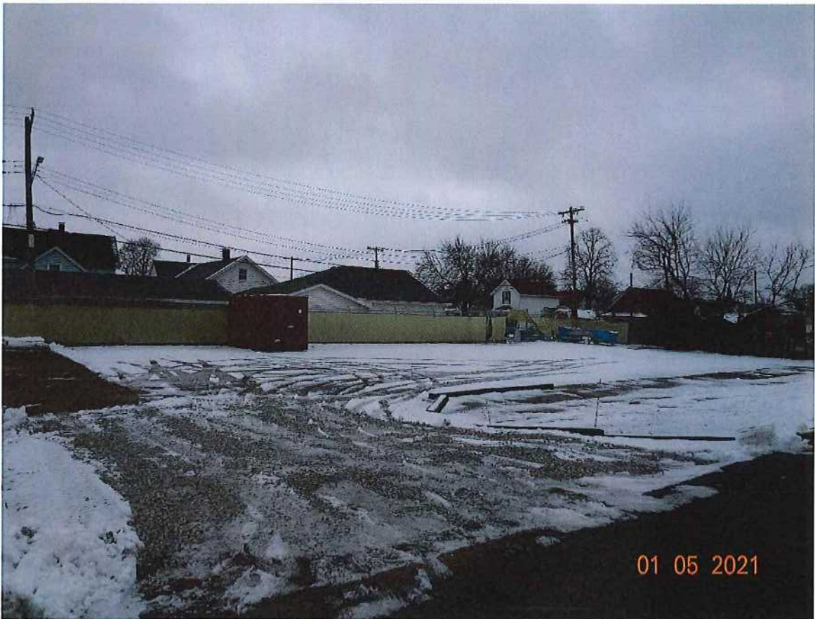
Rear parking lot of 411 S Main. Gravel to be removed or made hard surface.
