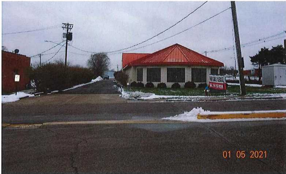
Front view of 403 S Main
