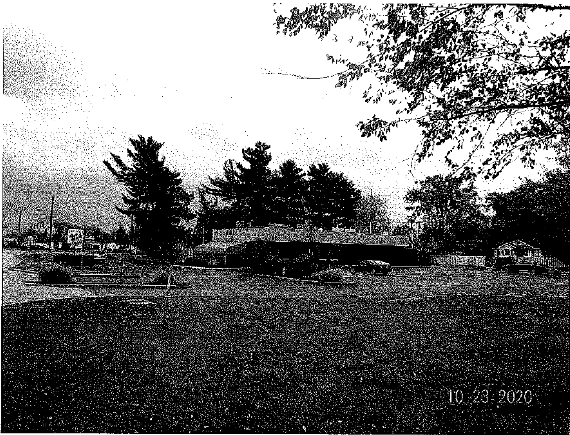
P4. Looking southeasterly toward the existing restaurant from the northwest corner of the site.
