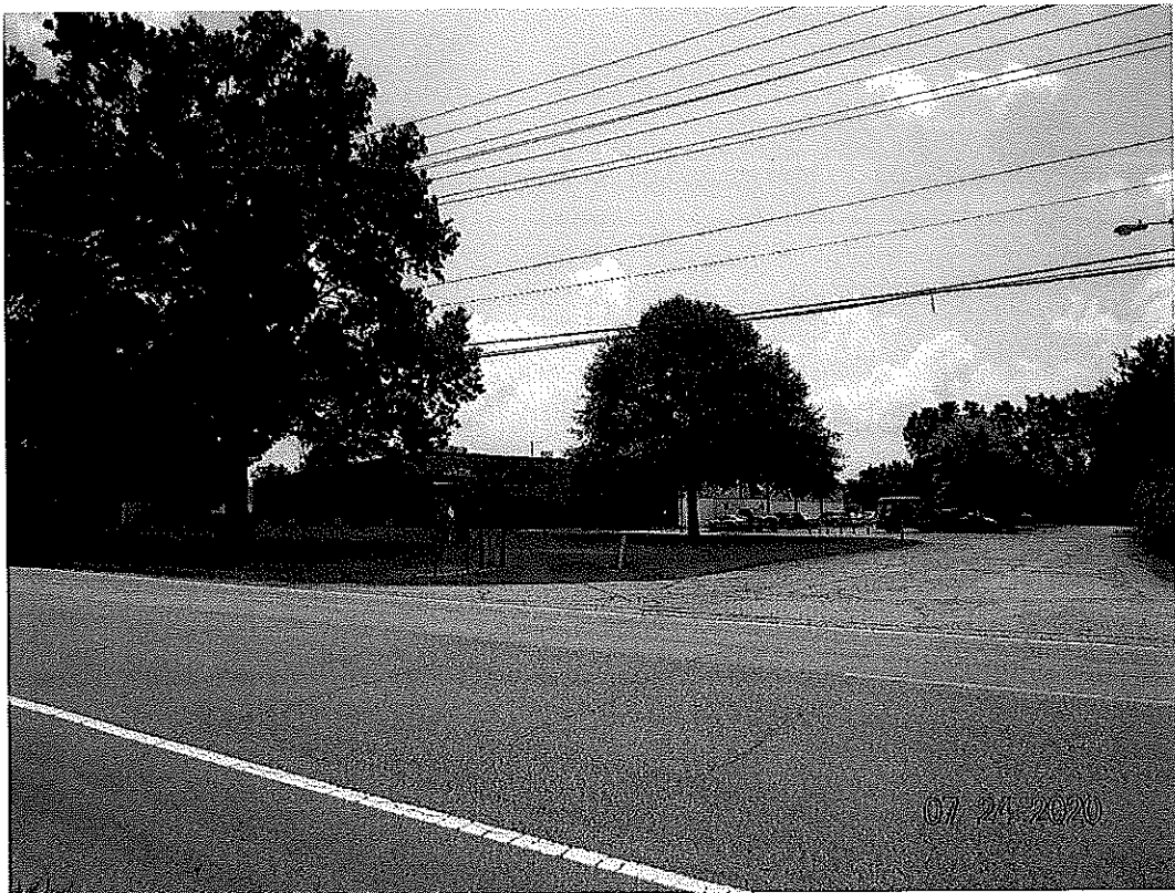
The Building at 1141 E Twelfth (annexation Parcel 2 south of parking lot).
