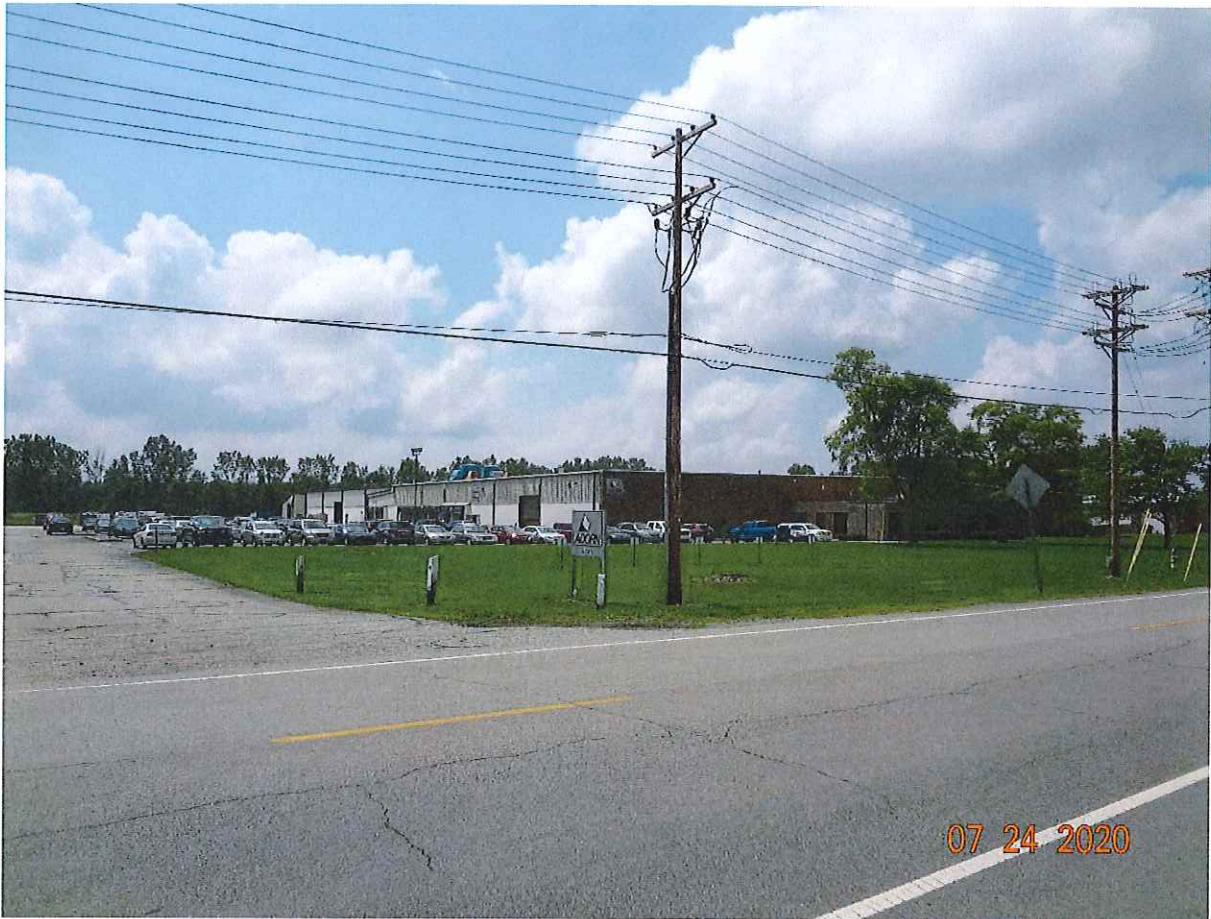
The building at 1241 E Twelfth (annexation Parcel 1 east of parking lot).
