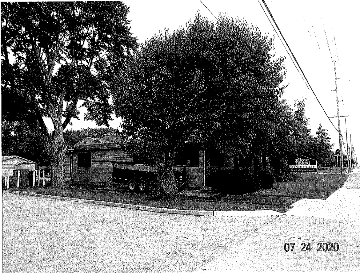
P3. Looking northerly from Grape Road toward the existing office building on proposed Lot 1.
