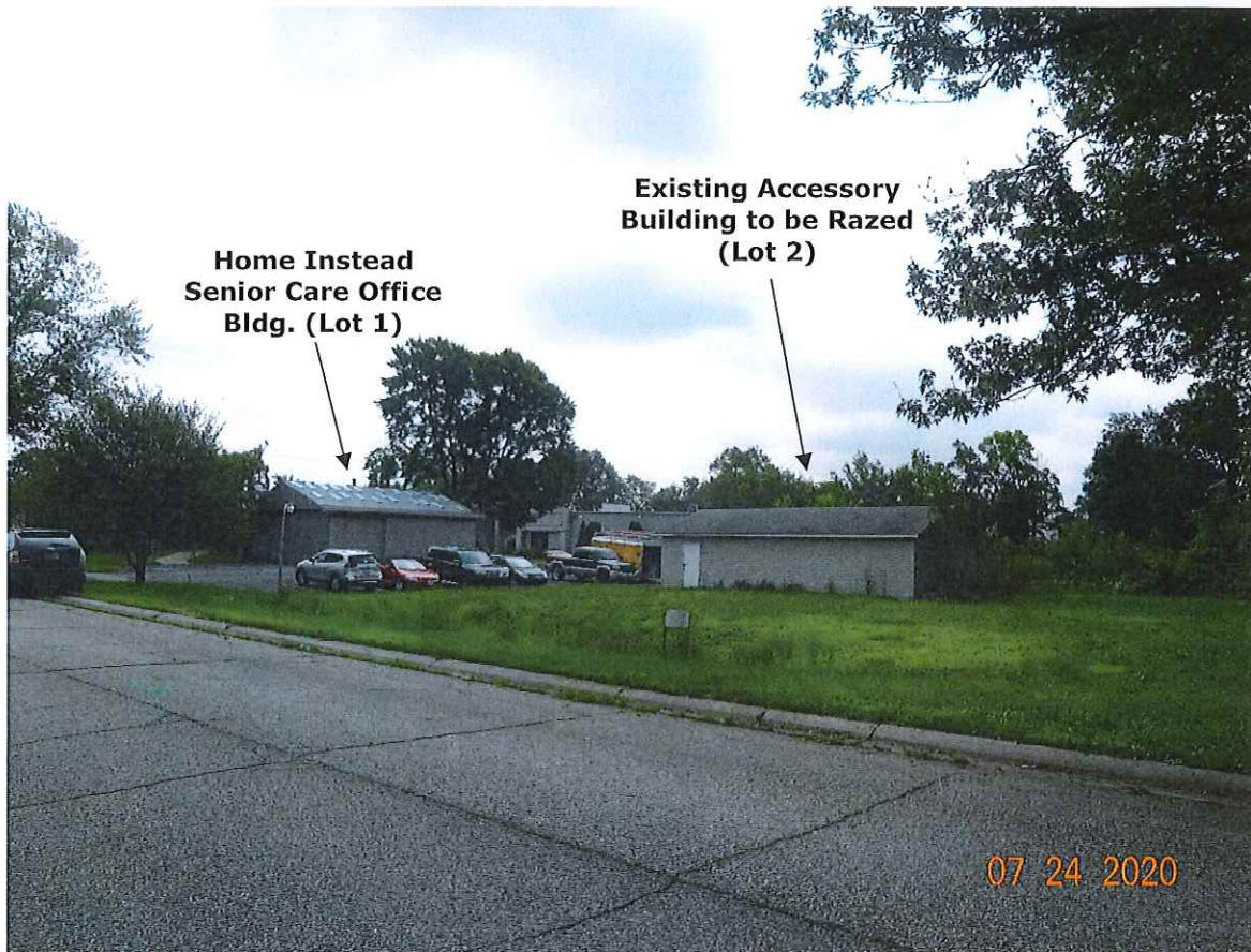
P1. Looking southeasterly from Eisenhower Drive toward proposed Lot 2 and the future location of a 6-unit senior care facility.
