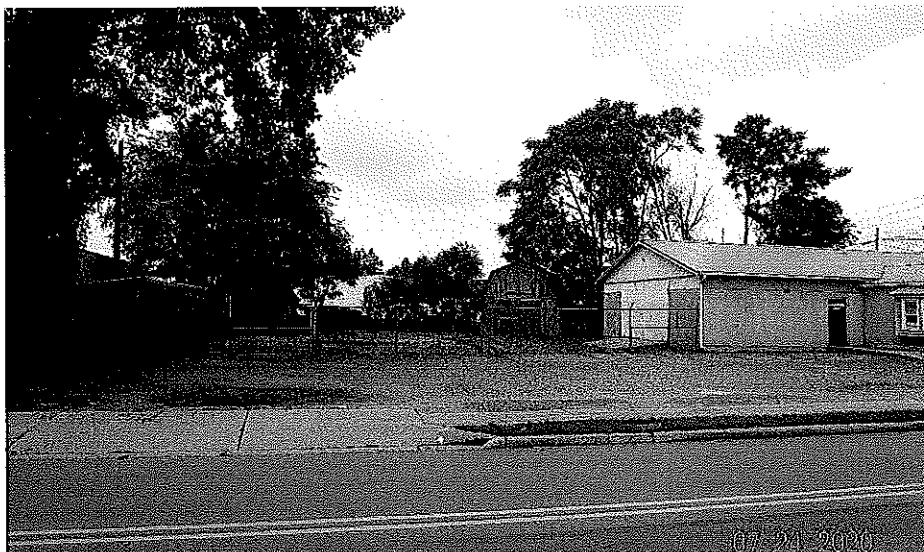
Rear storage area
