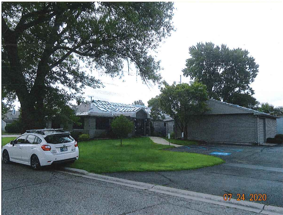
P2. Looking southeasterly from Eisenhower Drive toward the existing office building (Home Instead Senior Care) on proposed Lot 1.
