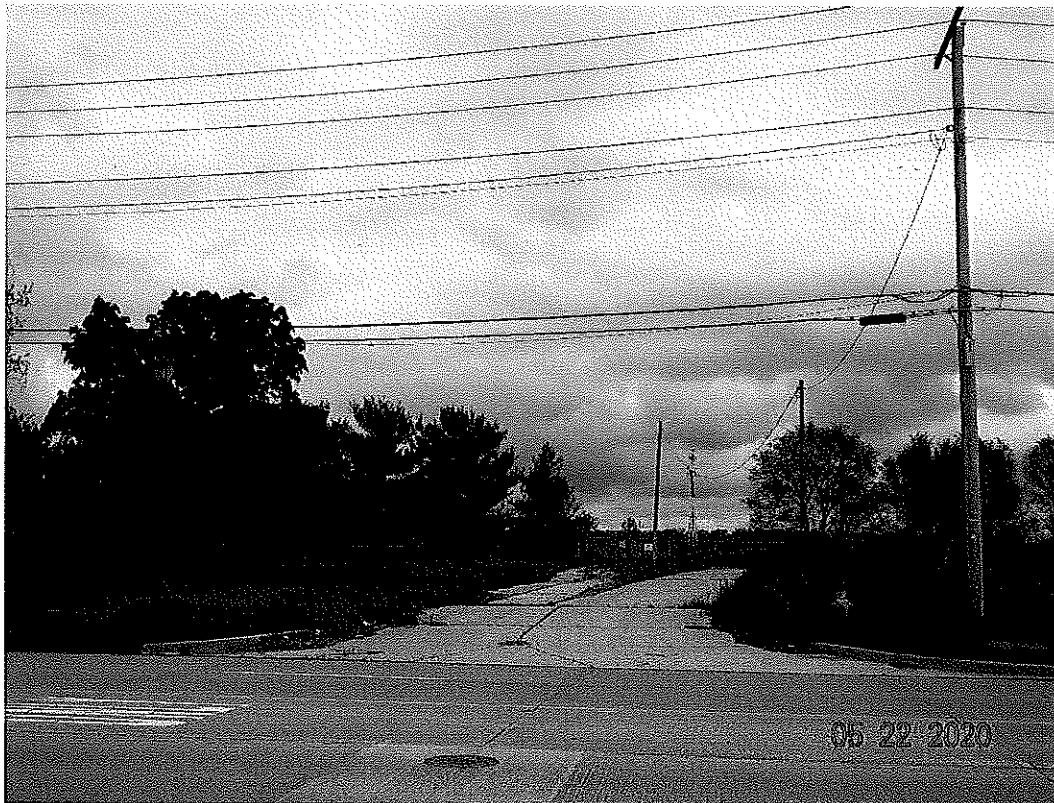
Looking northerly along the existing access drive on the east side of the annexation area.
