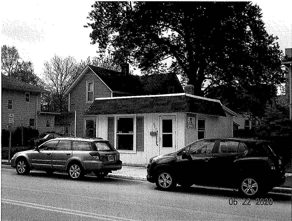
A view from Fourth Street in May 2020
