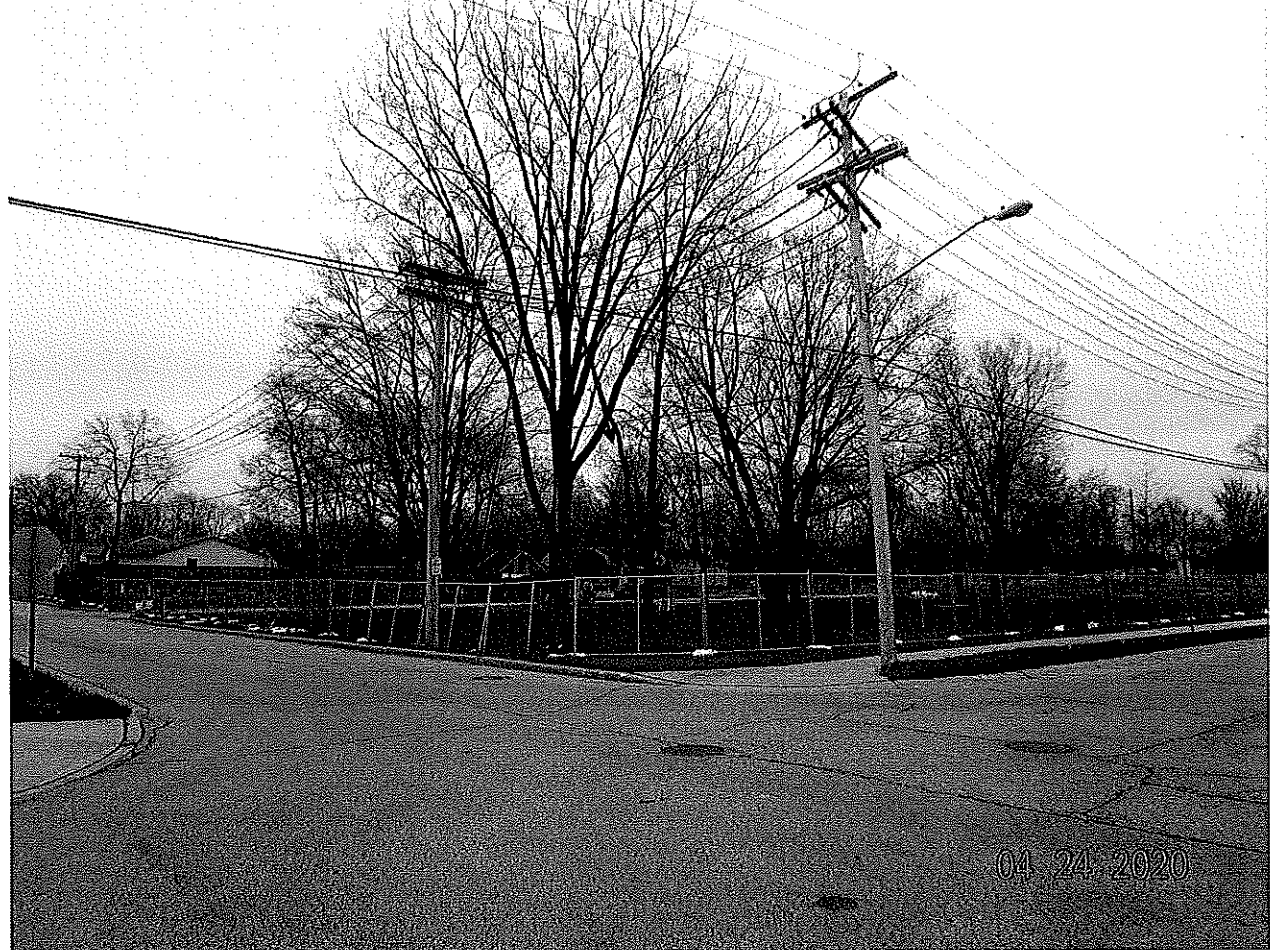
P1. Looking southeasterly toward the site from the W. Lowell Ave. & Clay St. intersection.
