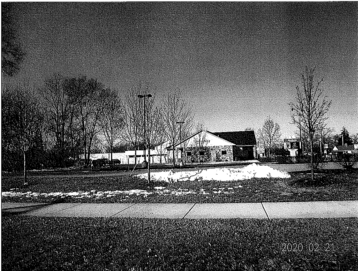
View of clinic looking west from Elder Road
