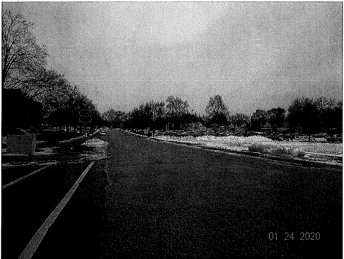
Looking south on Wenger Avenue
