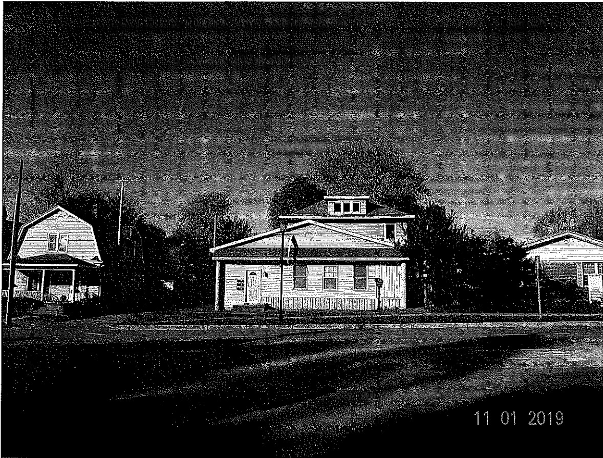
P3. Looking westerly toward the property from the east side of N. Main Street.
