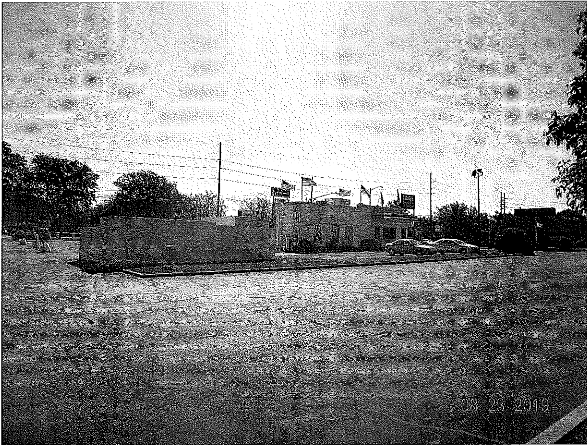
P4. Looking southeastly from the existing access drive to the west toward the property to be rezoned.
