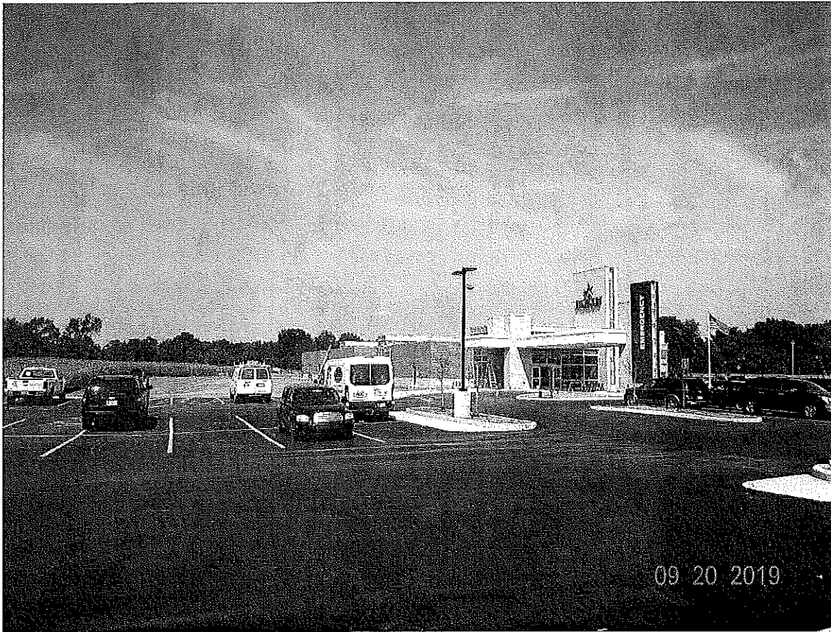
P1. Looking northwesterly toward Beacon Granger Hospital from the parking area to the southeast.
