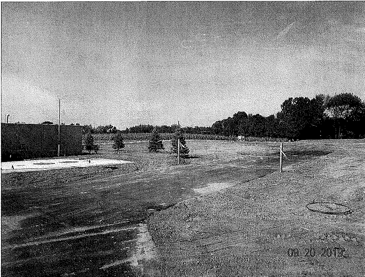
P2. Looking northwesterly toward the heliport from north of the hospital.
