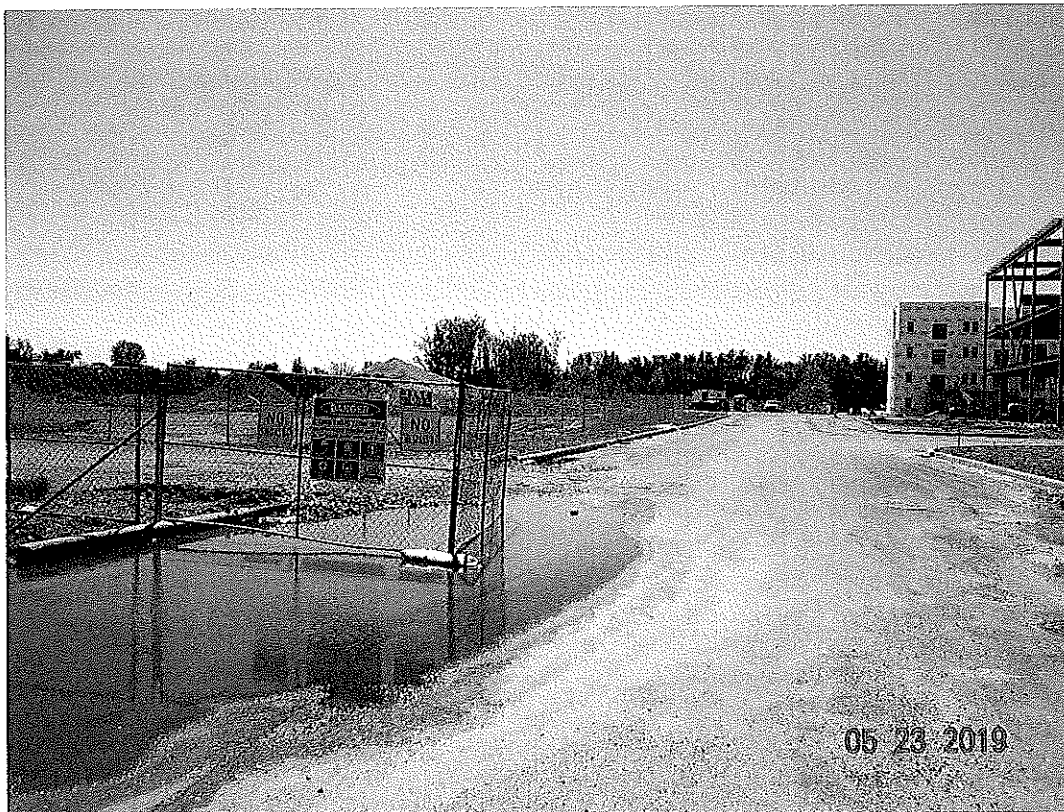
P1. Looking westerly into the site along Grandview Drive from Gumwood Drive south of Phase II of the Grandview PUD (currently under construction).
