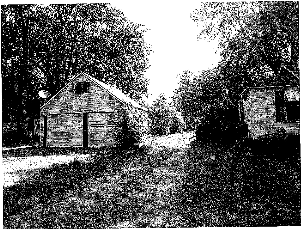
P2. Looking easterly down the alley south of the property.
