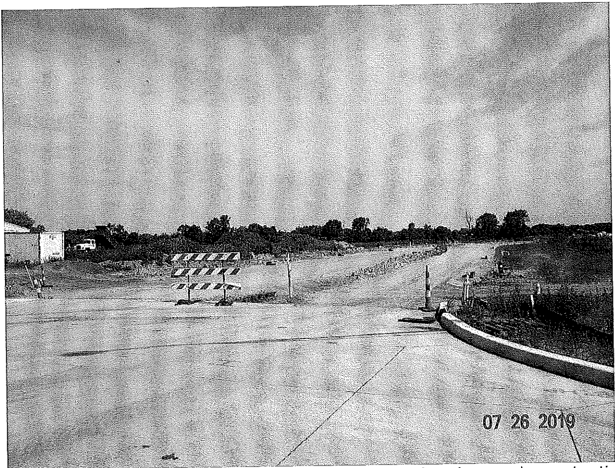
P2. Looking northerly along the east property line and Veteran's Parkway under construction.
