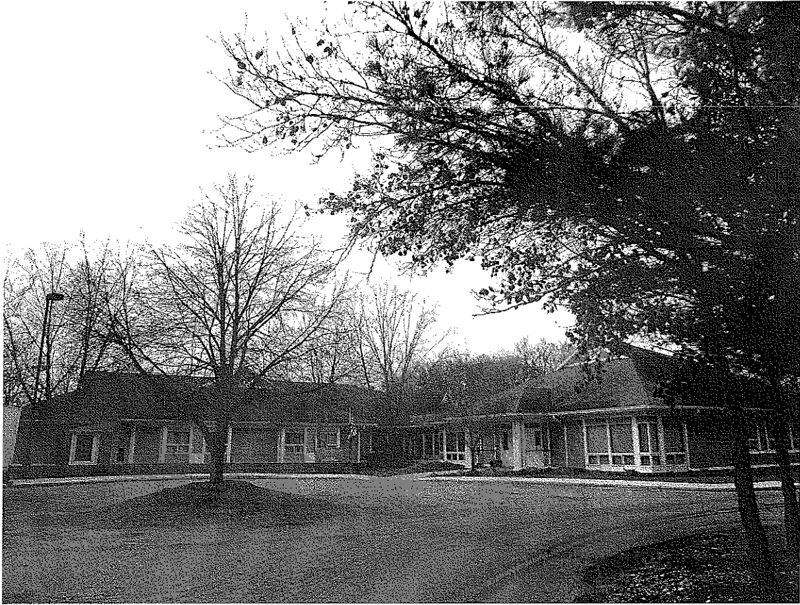
View looking onto existing hospital on site
