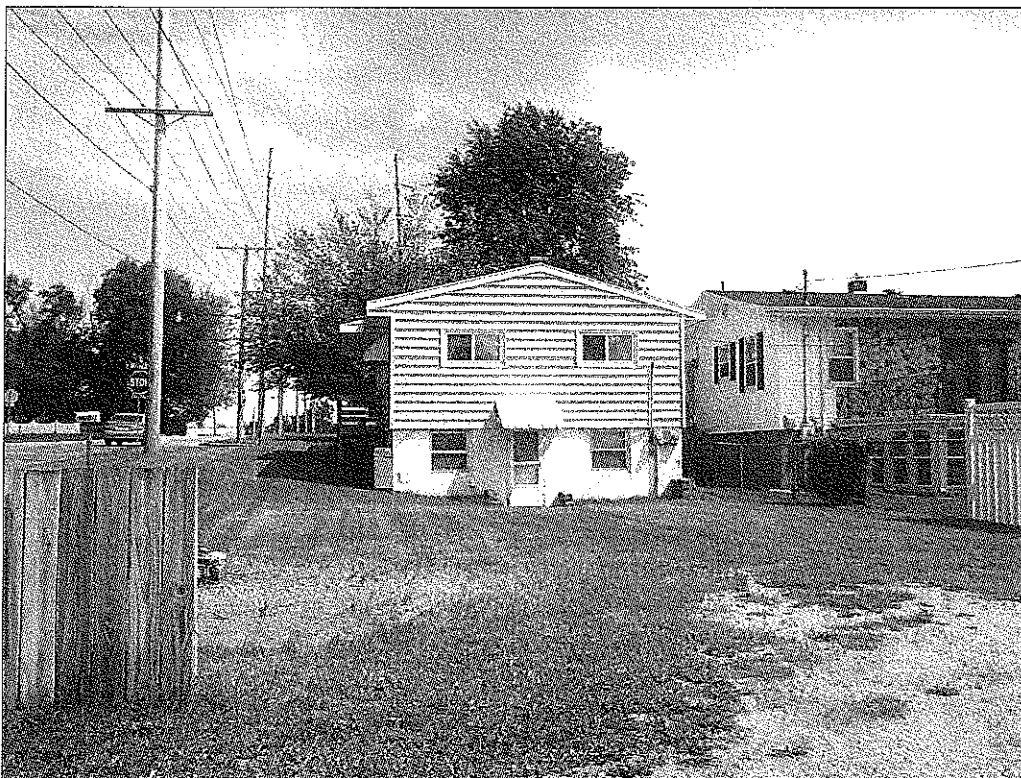
View of the rear of the home
