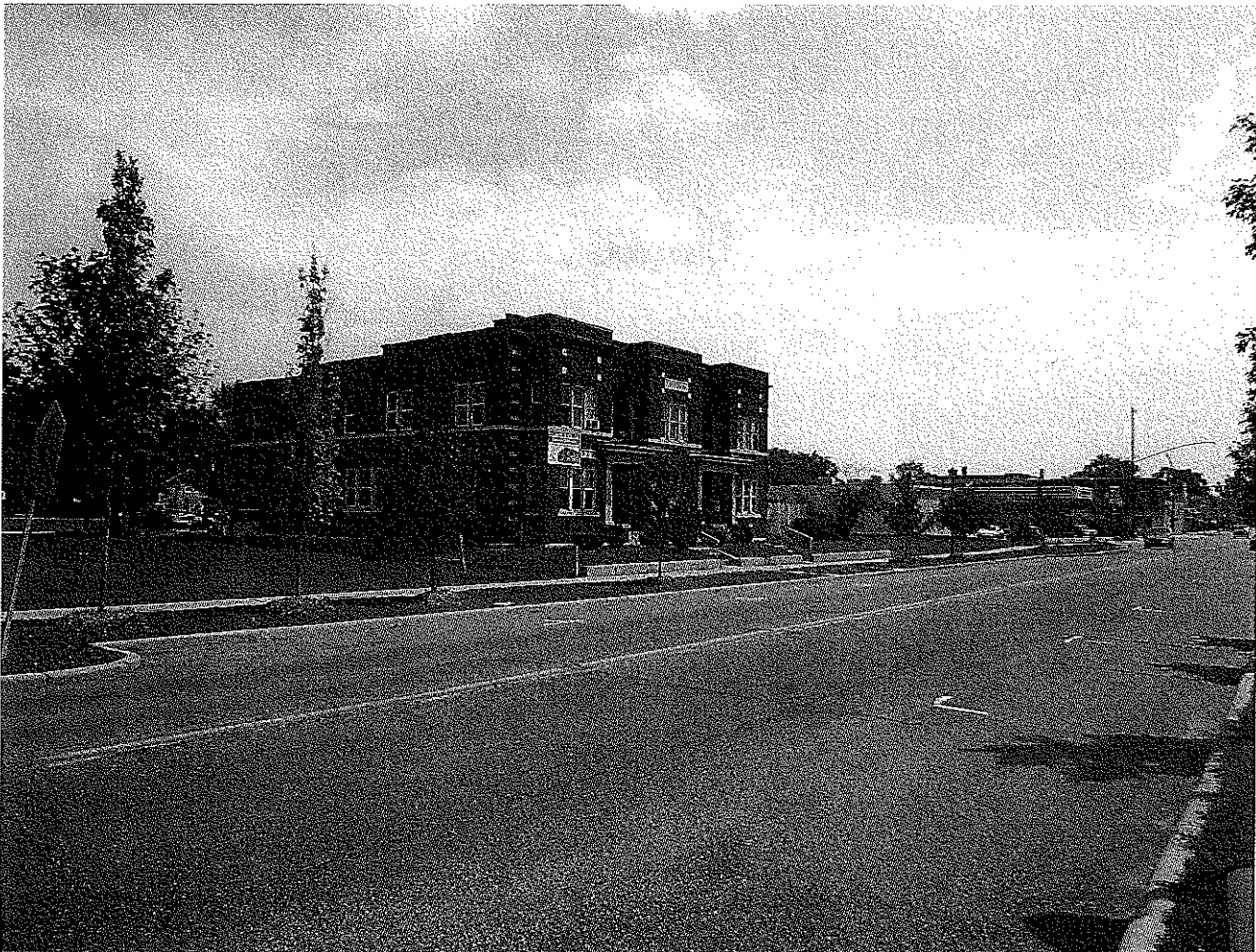
View looking northeast across Mishawaka Avenue from the Elizabeth Street intersection at existing apartment building to be demolished
