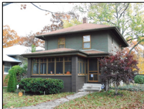
Award for Preservation Brian Finch and Bill Hawse Wilfred Dudding House 502 Calhoun St American Four Square c.1920 Notable #41067
