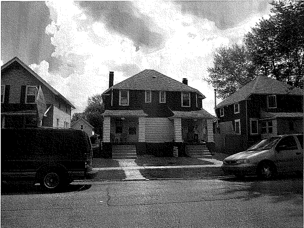
View of the Existing Duplex looking south from 11 th Street
