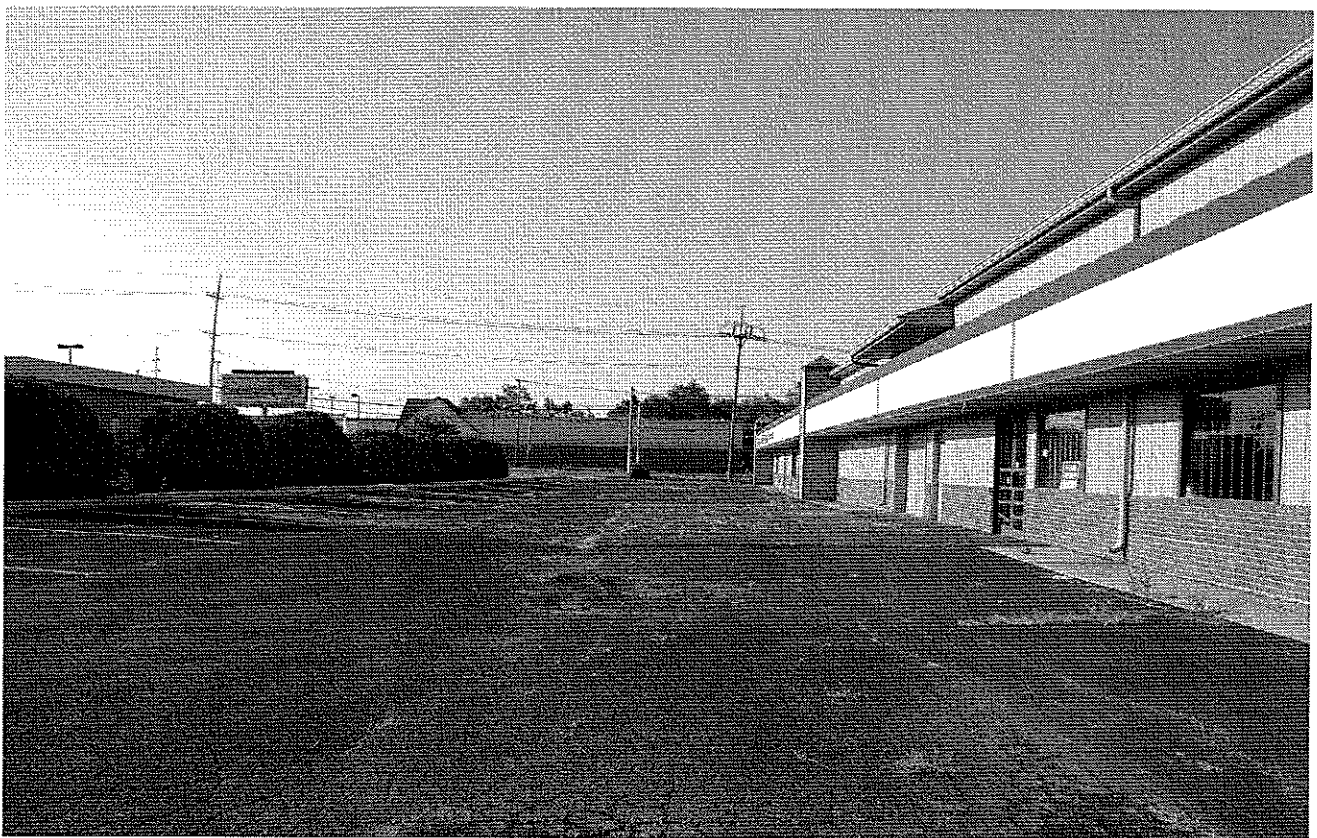
EAST SIDE OF BUILDING LOOKING SOUTH
