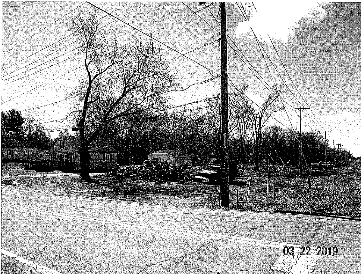
P1. Looking southwesterly from S. Elder Street and the railroad tracks toward the site to be rezoned.
