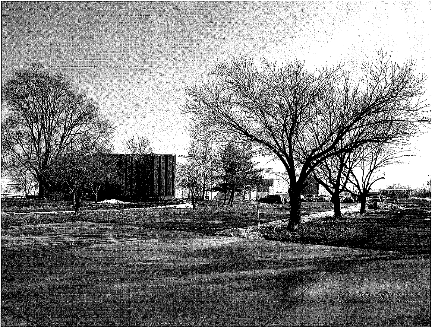
A view northeast from Byrkit Avenue of the building and parking area at 520 S. Byrkit Avenue.
