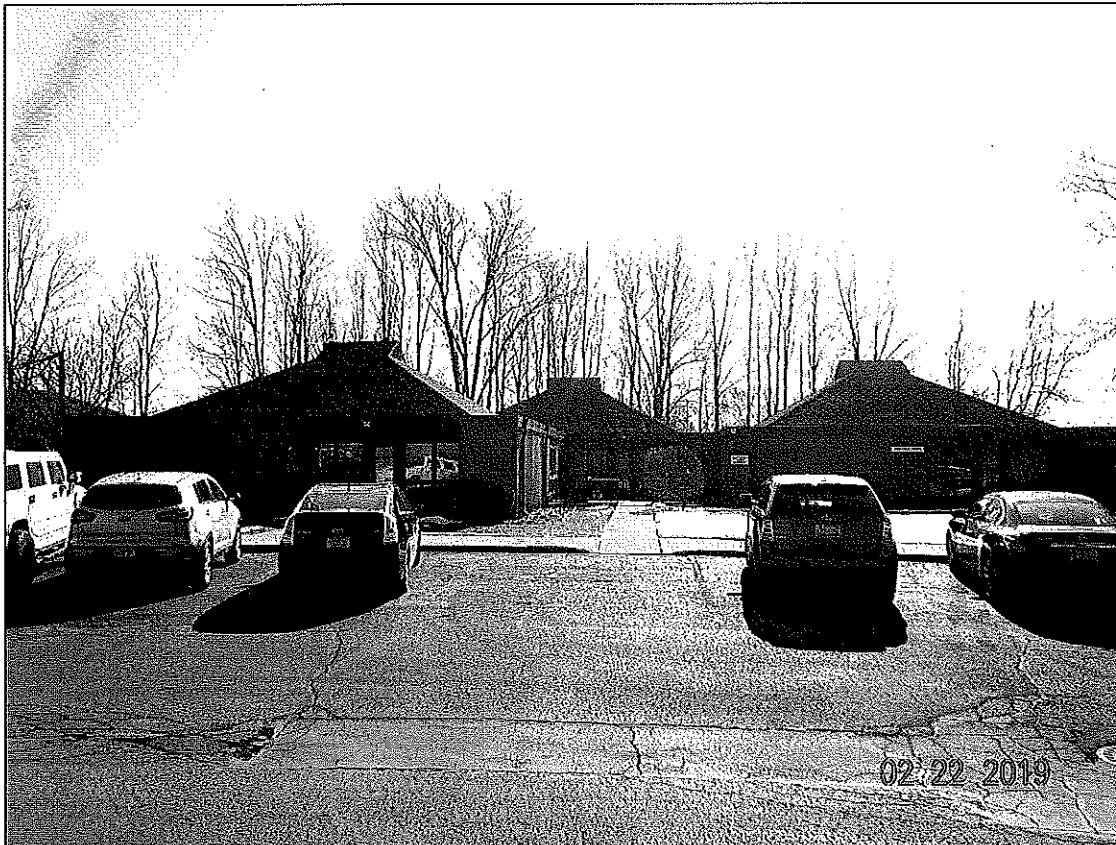
View of building
