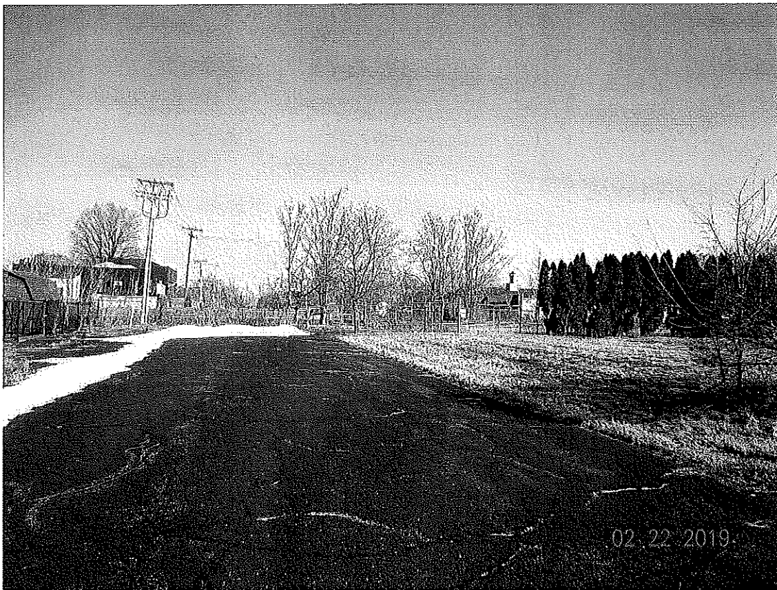
P2. Looking northern along vacated Union Street and the private drive to provide access to the site.
