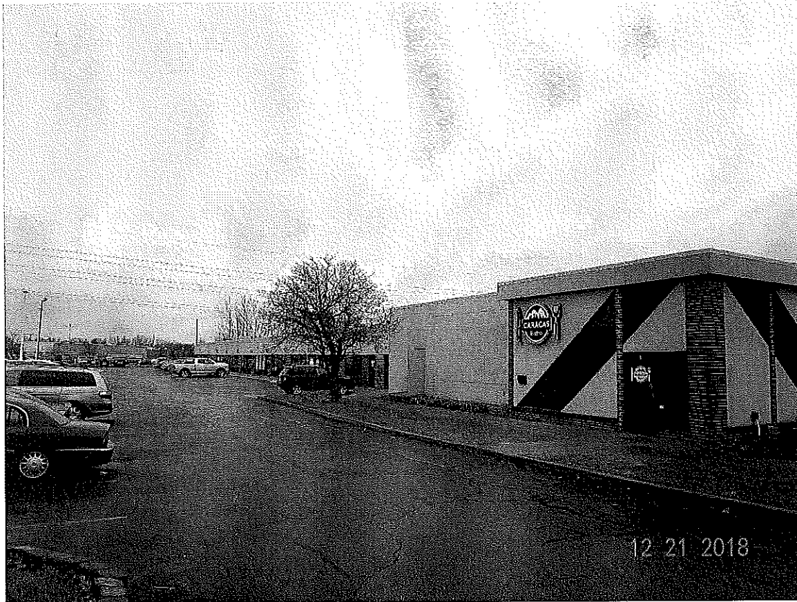
A view of the multi-tenant building from Edison Road
